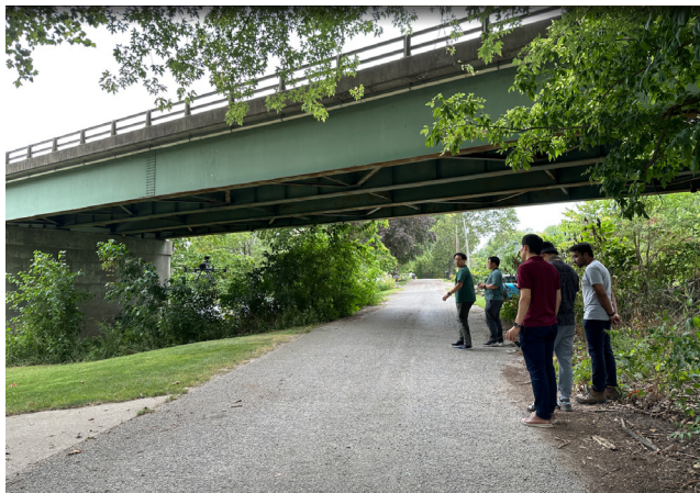
Figure 3.18 Summary of Field Implementation Testing Results at Davis Ferry Road Bridge. Target and Surroundings.
