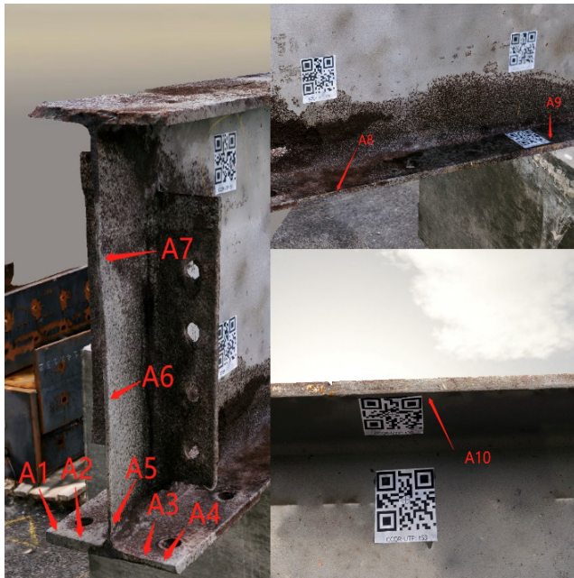
Figure 3.5 Measurement Locations and QR Code Targets on the Steel Girder.
