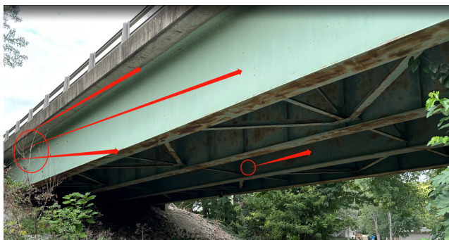
Figure 3.8 Outside W-section is Brighter Than Inside W-Section Due to Different Light Conditions.
