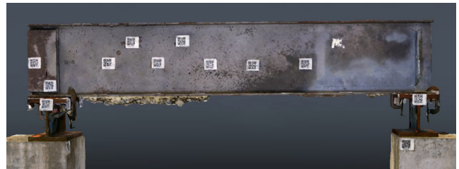
Figure 3.17 Vertical Views of the Resulting 3D Models. Scanning Date: August 10, 2023, Refined Sparse Capture Strategy.
