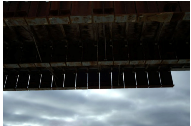
Figure 3.22 Incorrect Exposure and Resulting Incomplete 3D Model Sections: Incorrect Exposure Picture.
