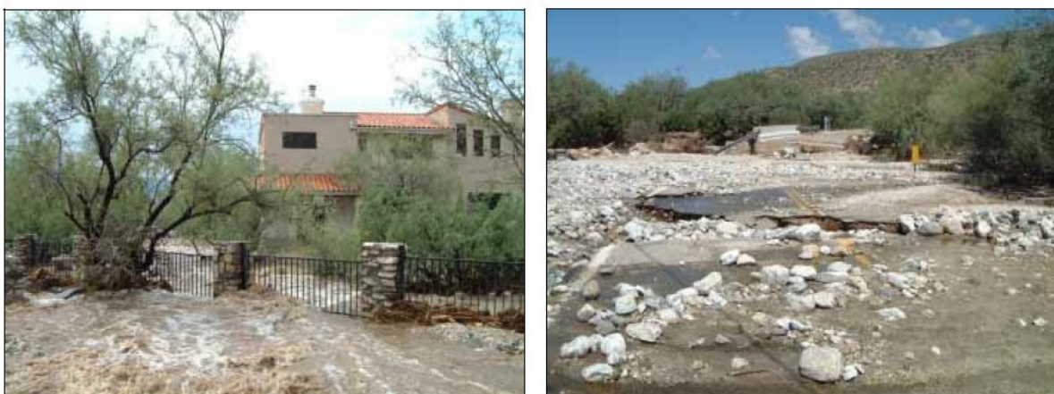
Figure B.27 Examples of a large flood event in an ephemeral stream that damaged roads, bridges, and flooded nearby homes in Tucson, Arizona, July 31, 2006 (Levick et al., 2008)
