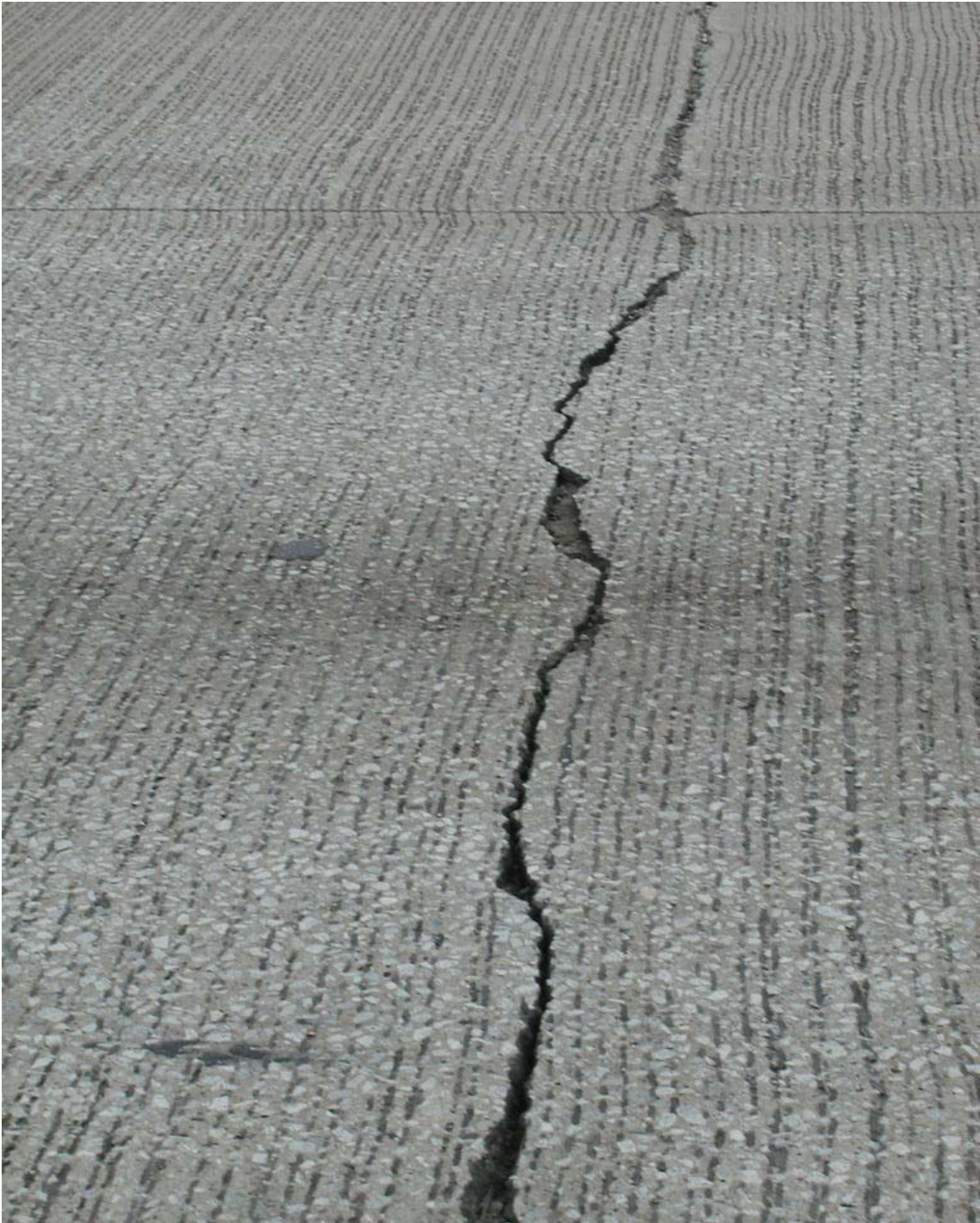
Sealed Crack in Concrete Pavement – Joint material seals the crack.
