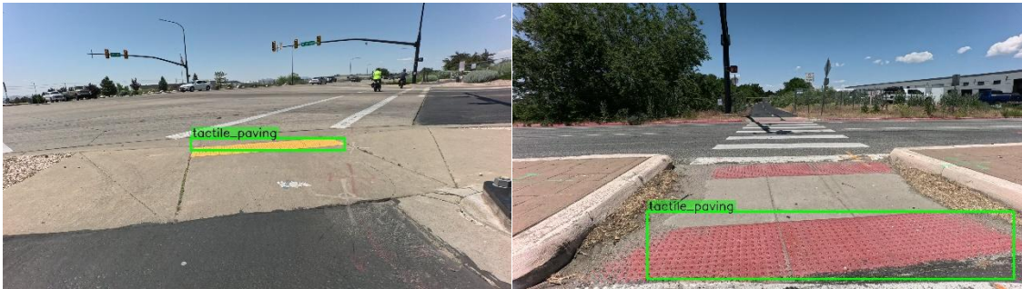
Figure C- 9: Tactile Pavement
