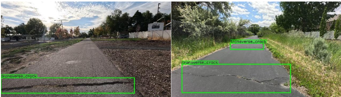
Figure C- 2: Transverse Crack
