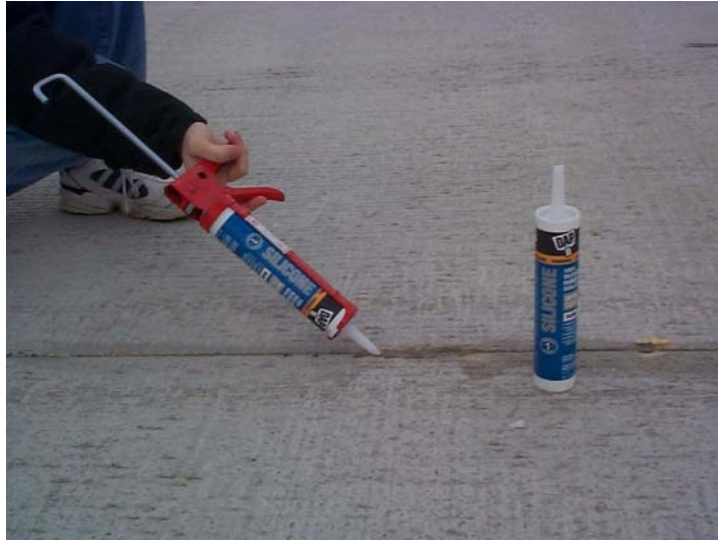
Figure 6-10 Silicon Caulking Operation
