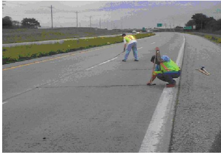
Figure 6-13 Sealant Removal Operation
