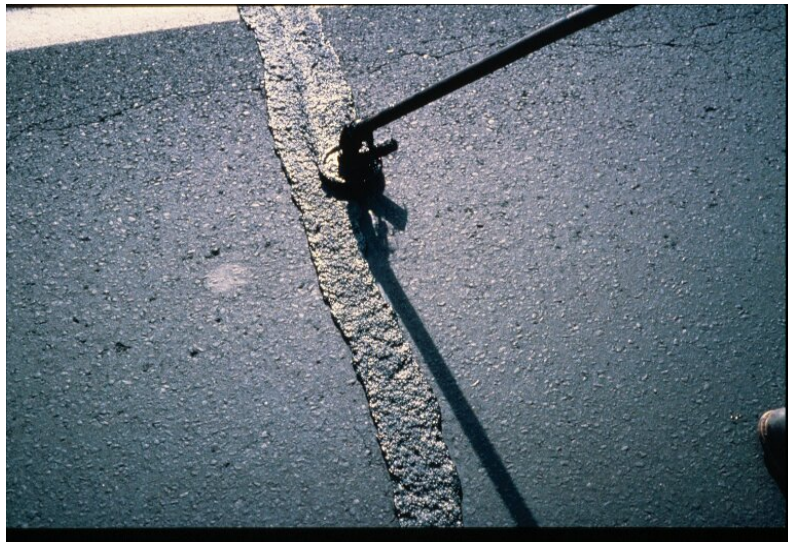
Figure 6-8 Sealing an HMA Pavement Crack
