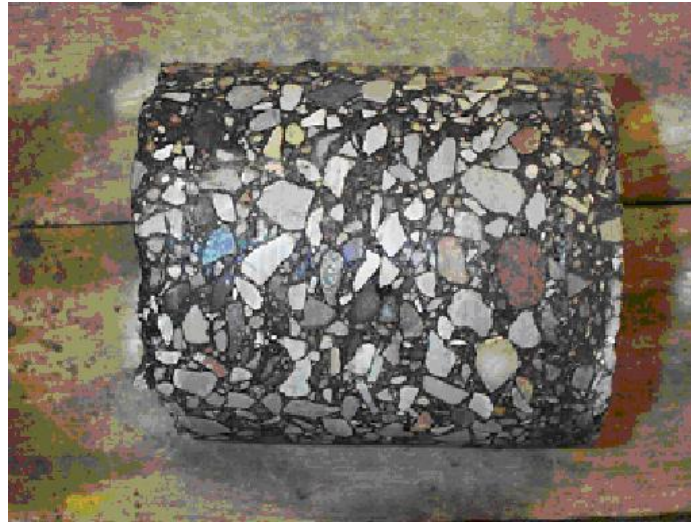
Figure E-1 Pavement Core on Northbound SR25
