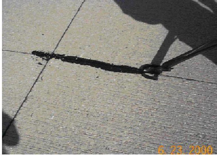
Figure 6-9 Sealing a PCC Pavement Joint
