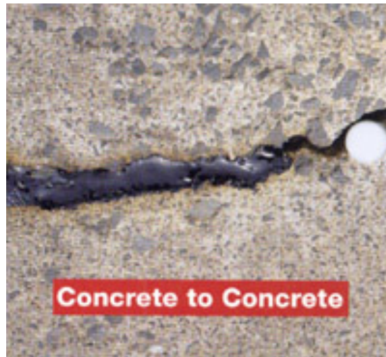
Figure 6-12 PCC Crack Sealed by Stix
