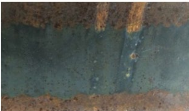
(a) Oxide layer in 2012 rail
