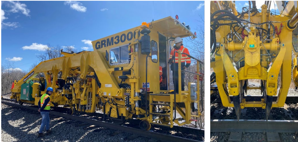
Figure 2. Plasser GRM3000T tamping machine
