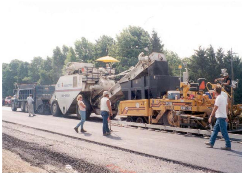
Figure 3.14 -- Pavement laydown operation
