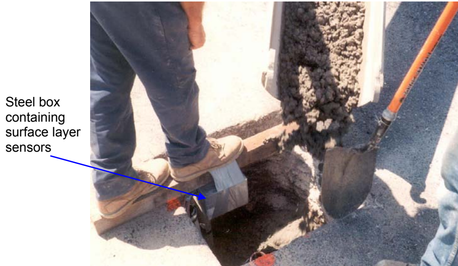
Figure 3.18 -- Backfilling the instrumentation pit with PCC
