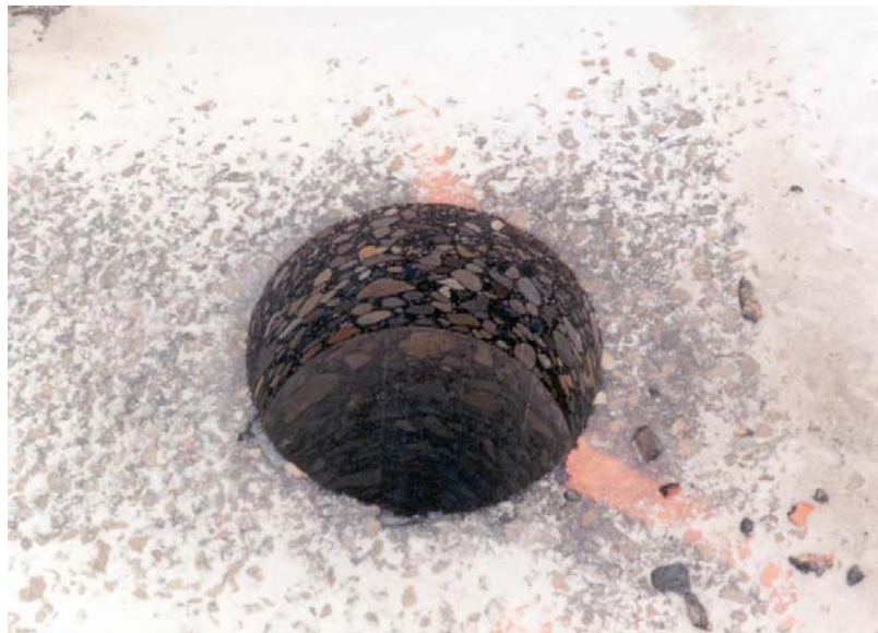
Figure 3.9 -- Hole showing pavement cross-section
