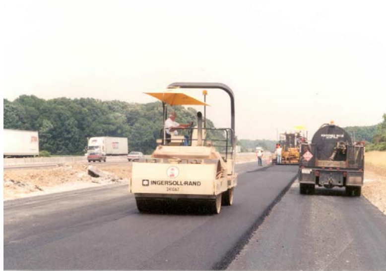
Figure 3.15 -- Pavement compaction operation
