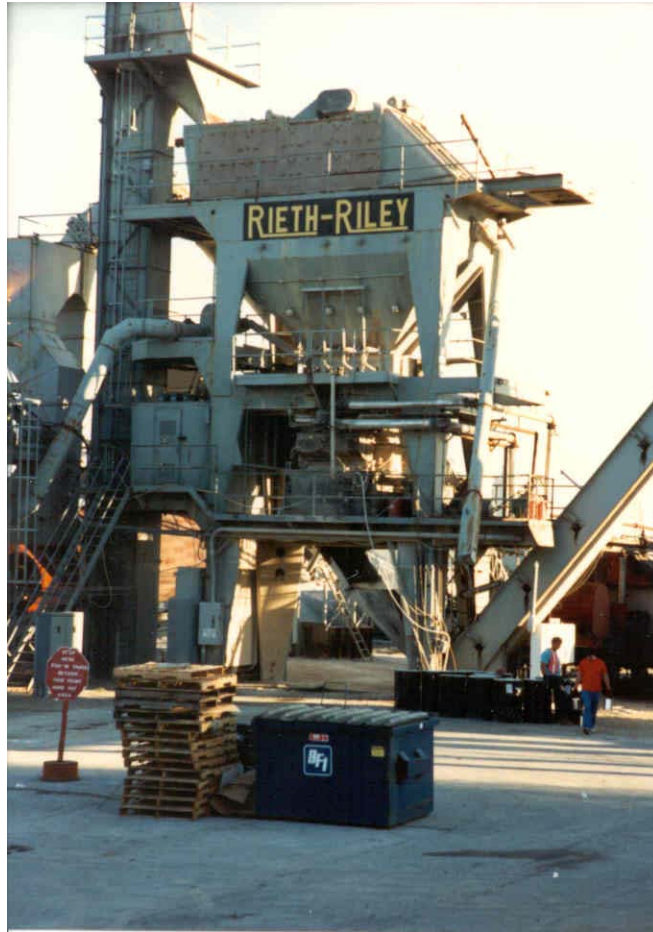
Figure 7 Hot Mix Batch Plant Used on Project
