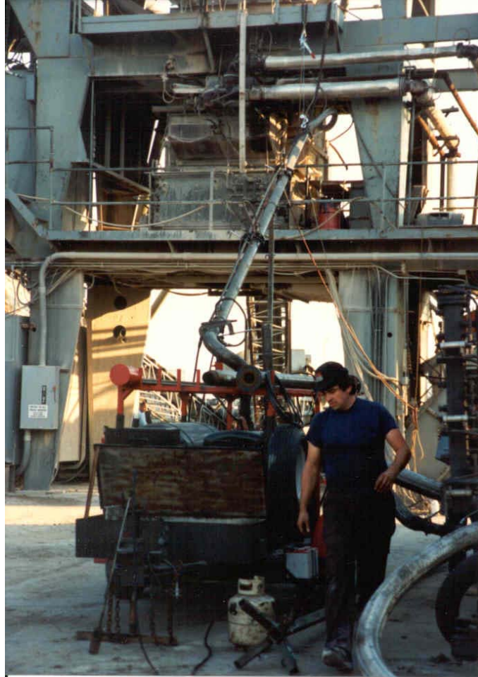
Figure 16 Pumping Reacted Asphalt Rubber into Plant
