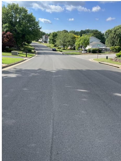
Figure 29. Photograph Taken 8 Months Post-Paving for Section with Mixture SM-9.5RPM P6 (State Route 1220). RPM = recycled plastic-modified; SM = surface mixture.
