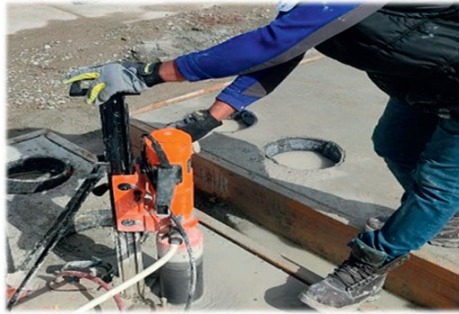
(d) Extraction of Concrete Cores From the Field
