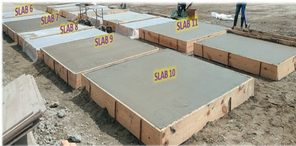
Figure 6.6 Overview of the Slabs Cast in the Field.
