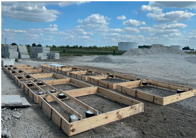
Figure 6.2 Assembled Formwork for Slab Casting.
