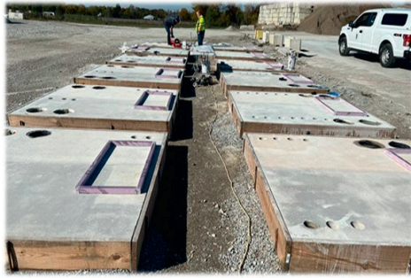
(a) Creation of Dikes on Field-Cast Slabs
