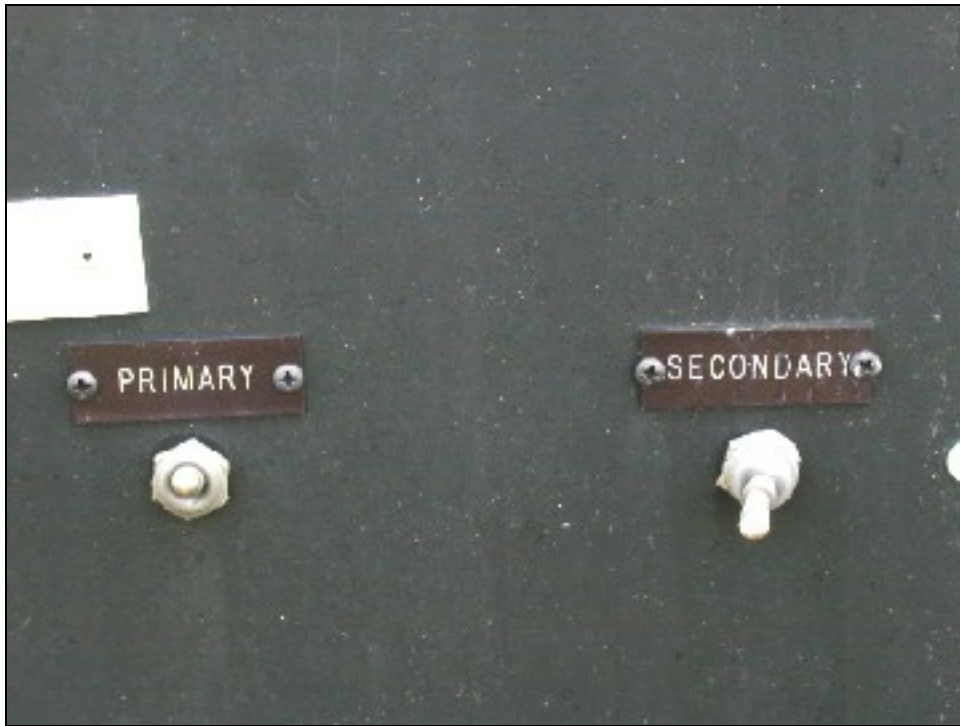
FIGURE A-5. ALTERNATE LAMP SWITCHES
