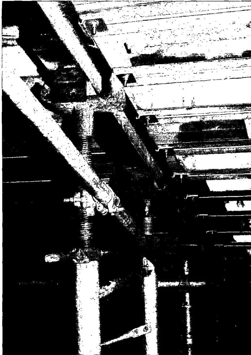
Figure 13. Bracing detail for screw leg supporting a sloped soffit.
