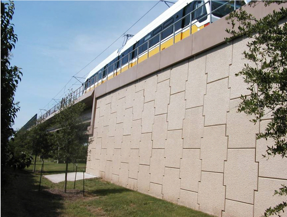
Source: Reinforced Earth Company
