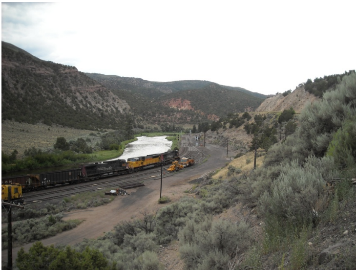
Exhibit 3-47: View west toward Dotsero along the UPRR
