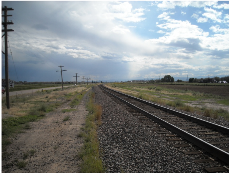
Exhibit 3-27: View south at UPRR MP 5.0, Sand Creek Junction
