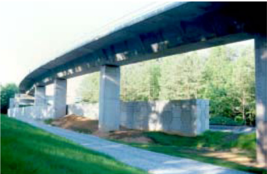
Source: Reinforced Earth Company
