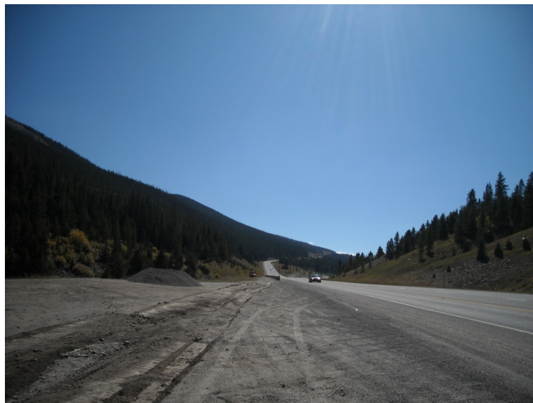
Exhibit 3-40: Typical condition of SH-9 and US-6 with space for guideway
