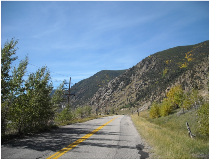
Exhibit 3-39: View of south of I-70 in vicinity of Georgetown
