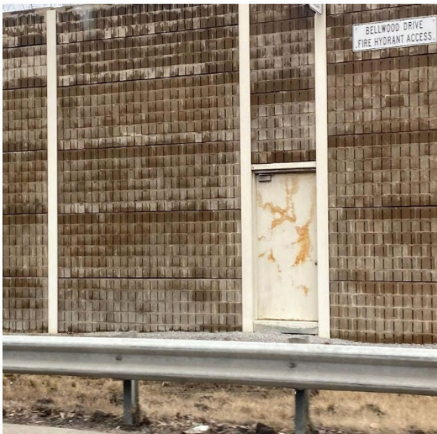
Figure 2.5 Noise Barrier With Fire Hydrant Access Door Along I-465.
