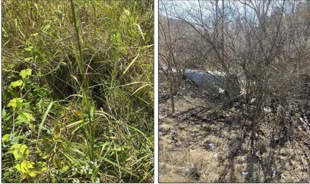
Figure D.4 & Figure D.5 Examples of culverts choked with vegetation along the Indiana ROW. These images were captured during culvert inspections. The culvert on the right is located approximately 100 feet from the road edge behind a noise barrier. Photos taken by INDOT staff, used with permission.
