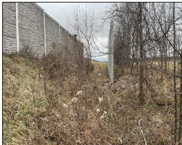
Figure D.8 Vegetation built up behind a noise barrier along I-65, Lebanon, IN.
