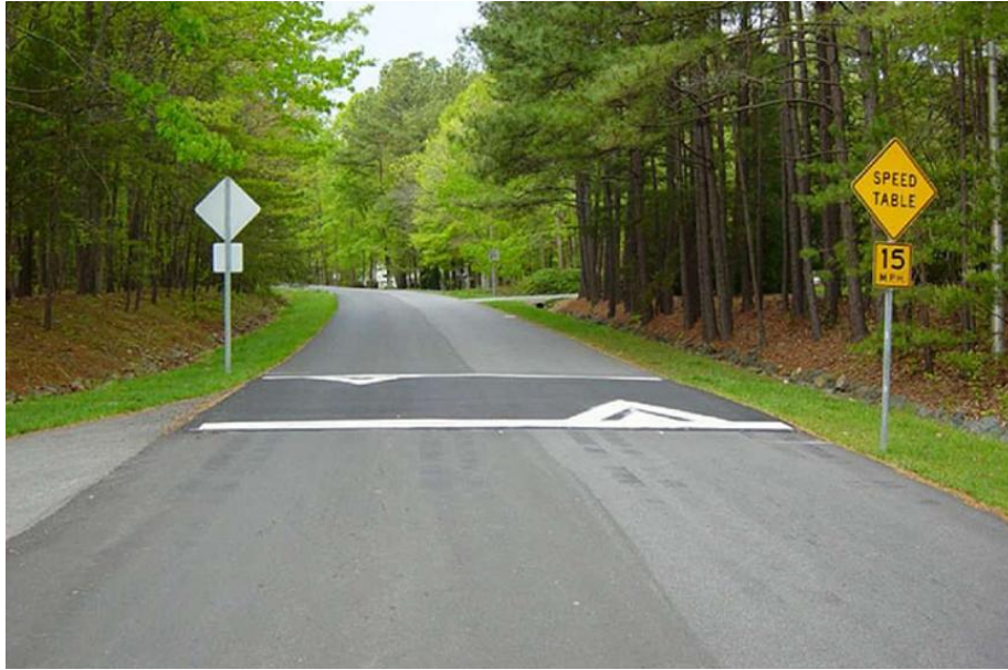
Figure 3.10 Speed Table (FHWA, 2018b)
