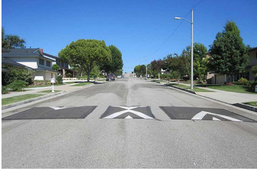
Figure 3.9 Speed Cushion (FHWA, 2018b)
