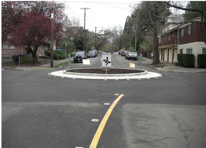
Figure 3.7 Traffic Circle (FHWA, 2018b)
