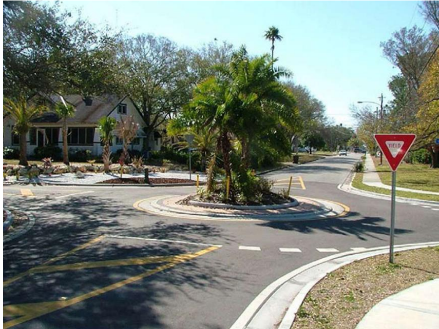
Figure 3.5 Small Modern Roundabout (FHWA, 2018b)
