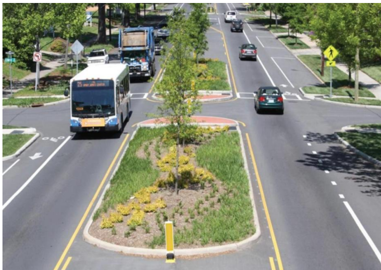
Figure 3.17 Median Island (FHWA, 2026c)
