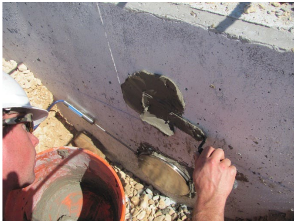
(c) Field installation of pressure cell.
