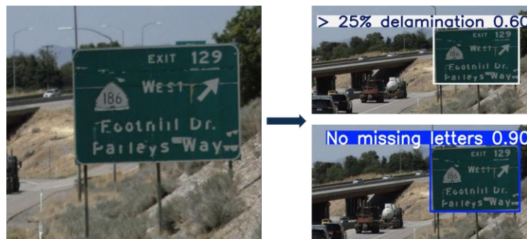
Figure 5.17: Co-existing delamination and missing letters defect
