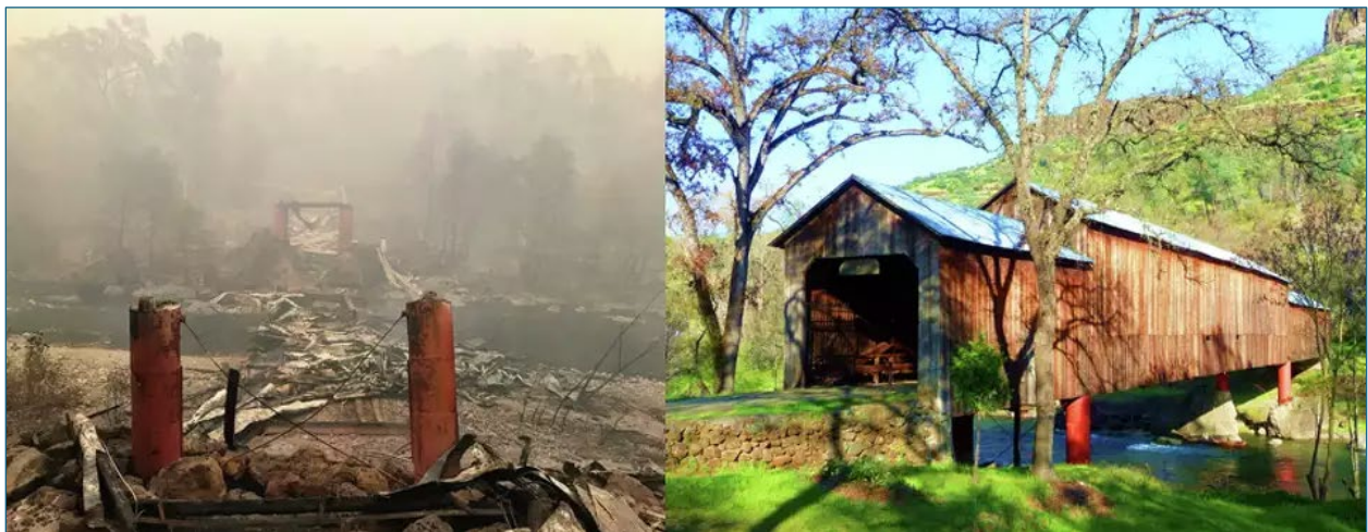
Figure 10. Photos. Honey Run Covered Bridge post-fire (left) and pre-fire (right) [122].
