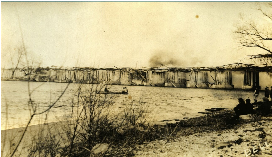
Figure 1. Photo. DeKalb Street Bridge post-fire.[66].
