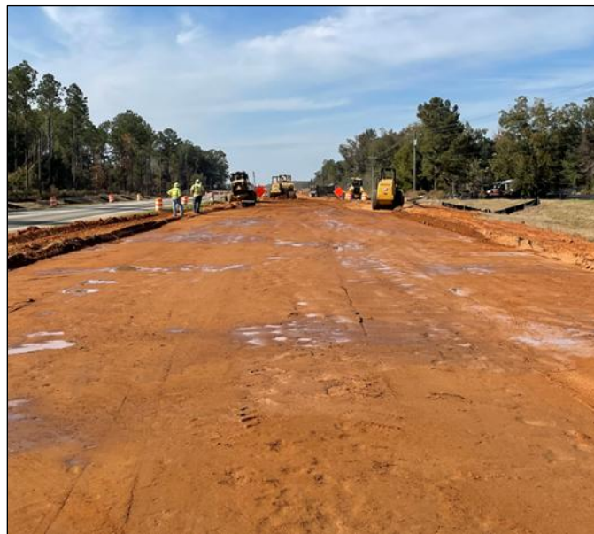
Figure 8. Photo. Compacted and wet soil-cement.
