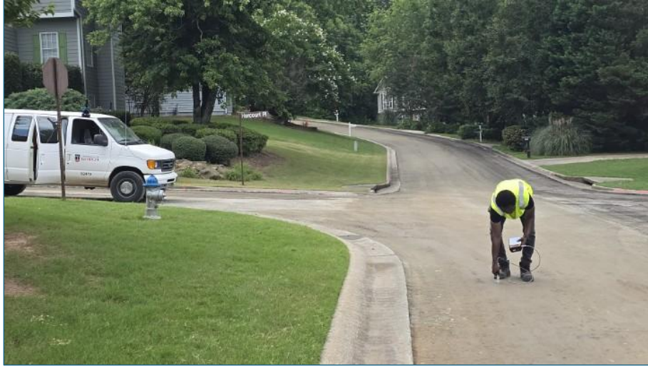
Figure 25. Photo. Percometer scanning of the stabilized road base.
