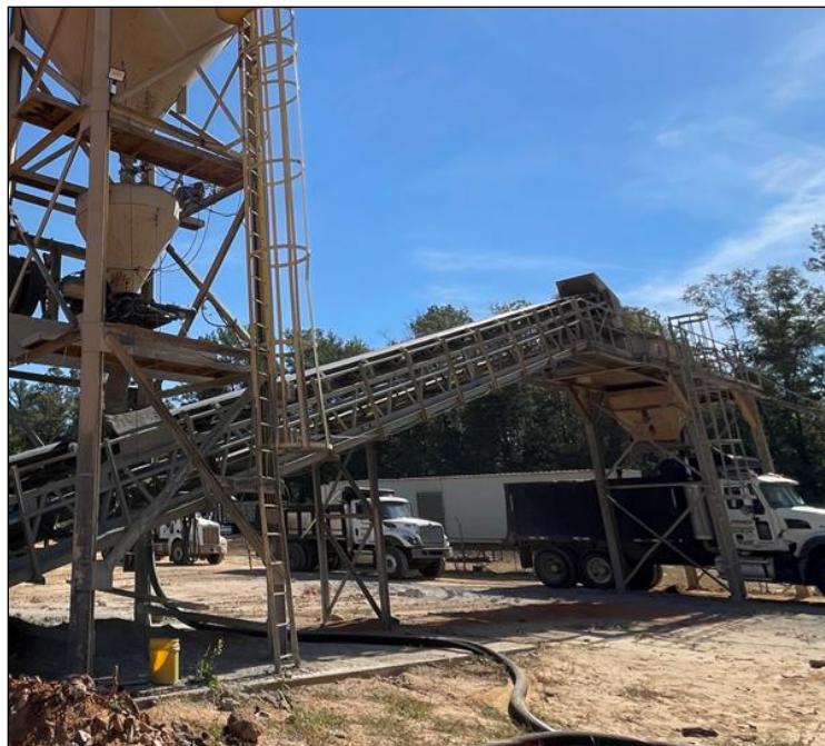
Figure 6. Photo. Soil-cement mixing auger at the plant.
