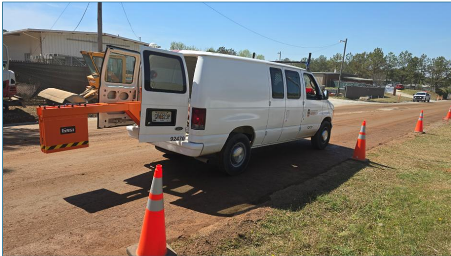
Figure 24. Photo. GPR scanning of the stabilized base.
