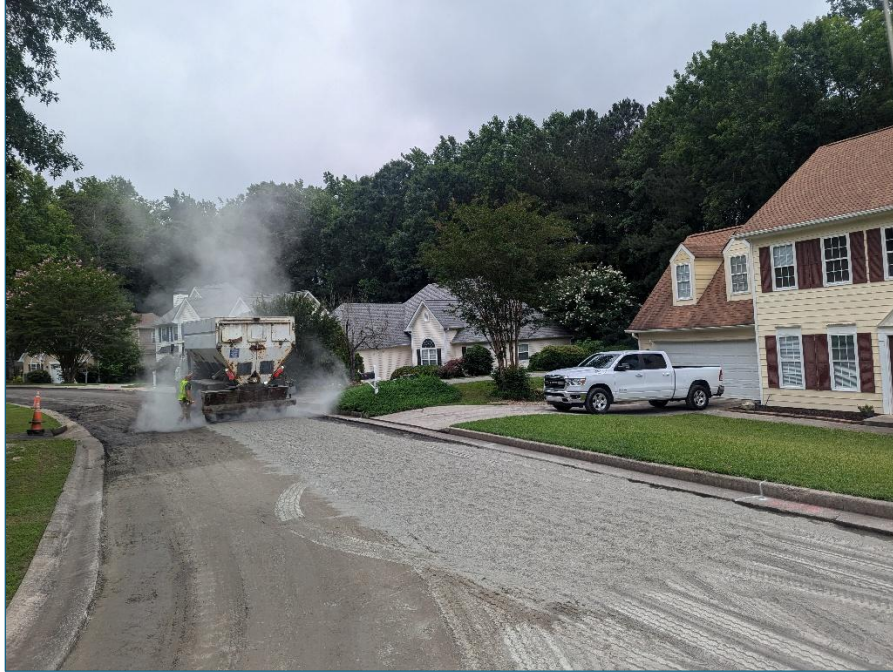
Figure 59. Photo. Application of cement with spreader truck.
