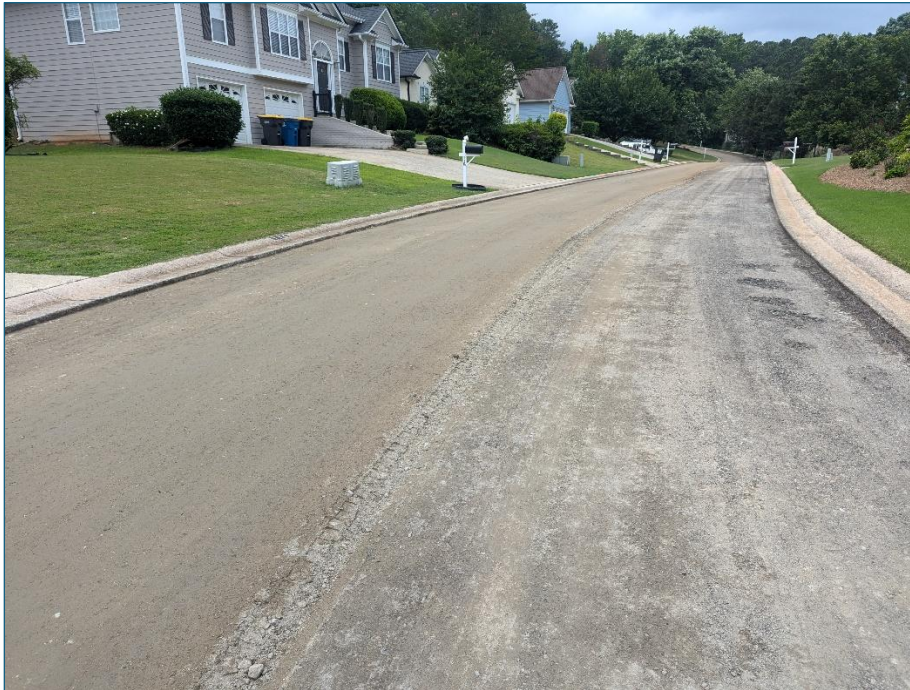
Figure 58. Photo. Milling the asphaltic layer.
