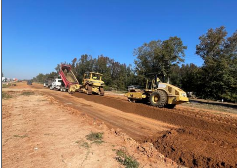
Figure 7. Photo. Jersey spreader, spreading the soil-cement on the construction site.
