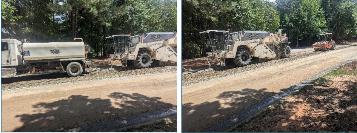
Figure 60. Photos. Reclaimer machine mixing cement with FDR base.
