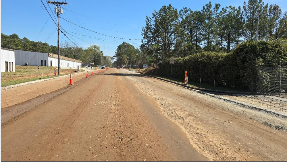
Figure 11. Photo. Stabilized FDR base at Old Covington Road.
