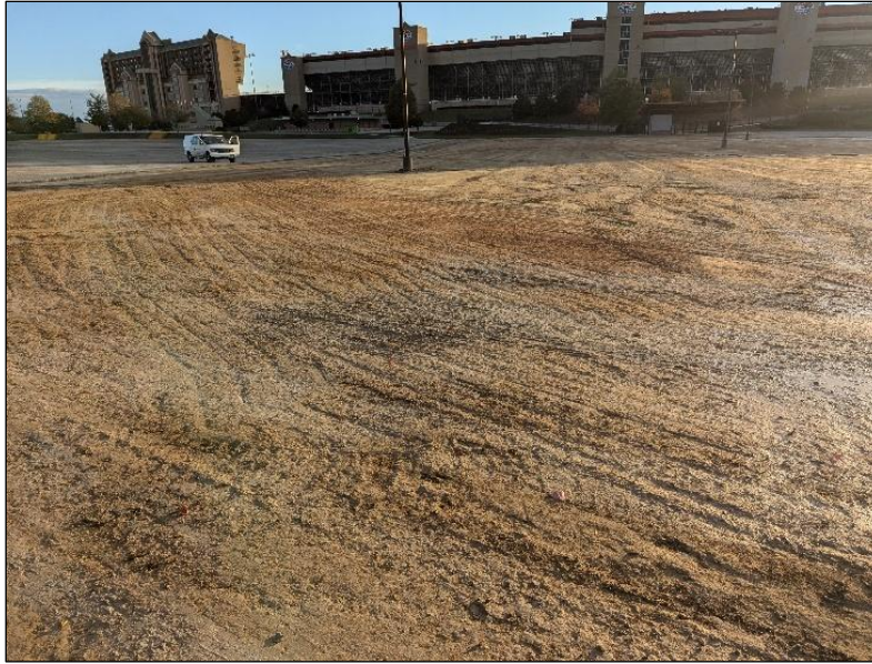
Figure 9. Photo. Stabilized FDR base at Atlanta Motor Speedway.
