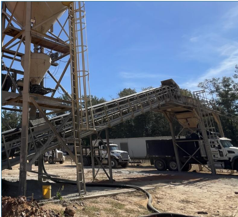
Figure 57. Photo. Soil-cement plant.
