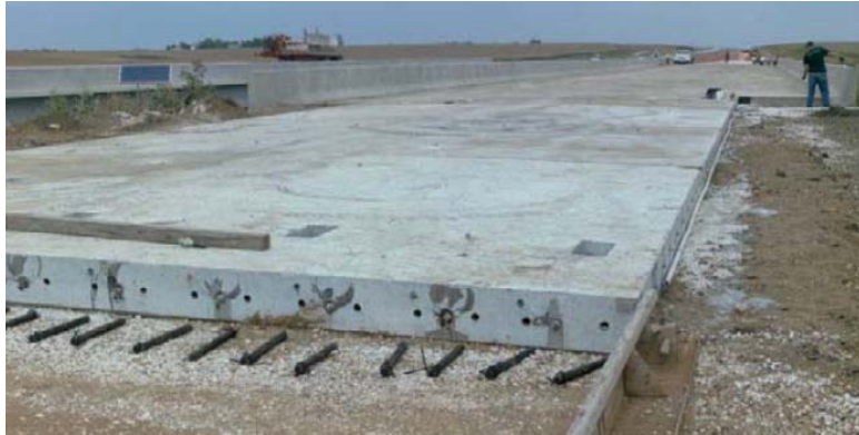
Figure 5-7 Epoxy-coated dowels to be installed at the BAS – pavement joint [11]
