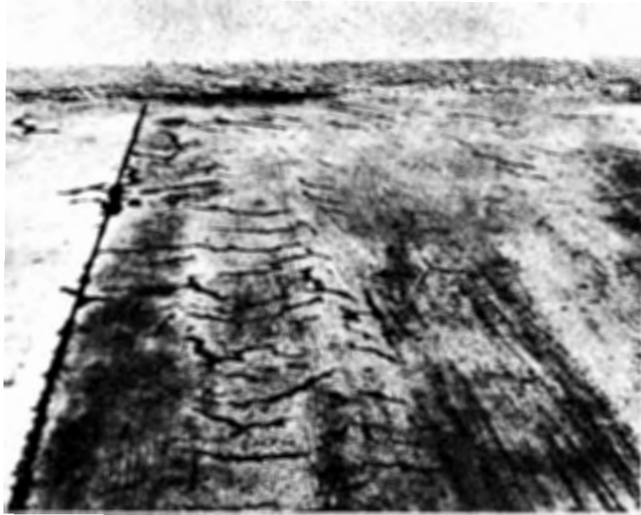
Photographs 25 & 26: Crack surveys were run on the deck both before and after heat treating.
