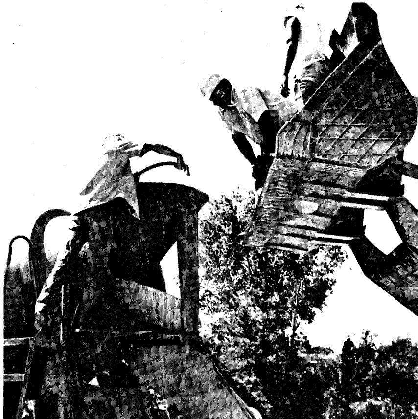
Photograph 4: Water was used to wash all of the beads into the drum.
