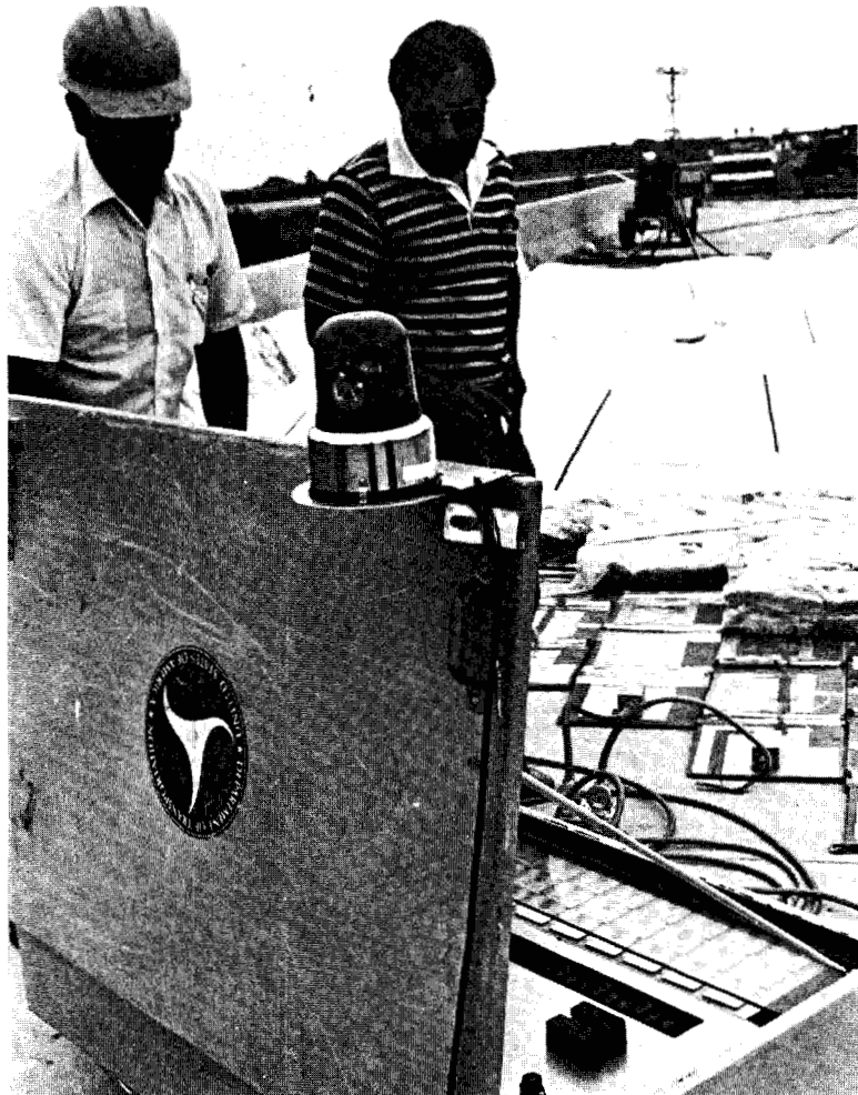
Photographs 15 & 16: Control console. Flashing red light would come on automatically if any of the circuits broke.
