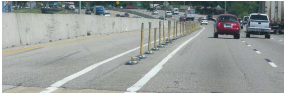
Figure 6- 1: Pylon at Merge and Diverge Area
