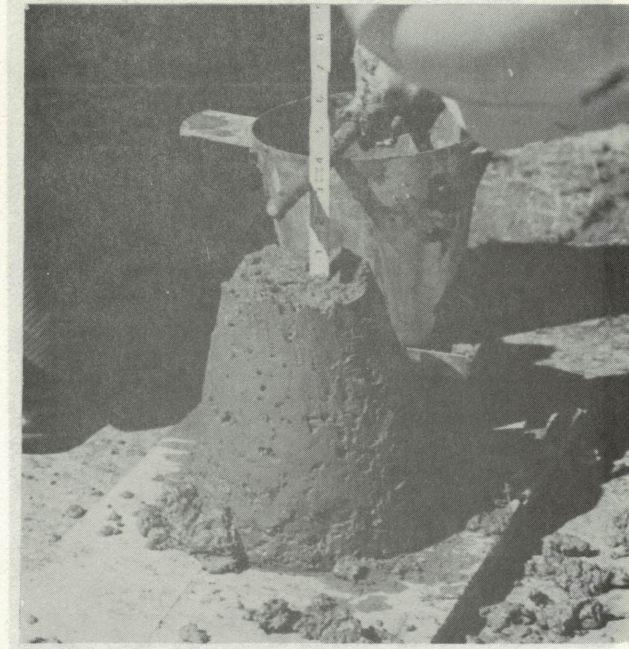
Figure 21: Inspector measures 3 inches of slump.
