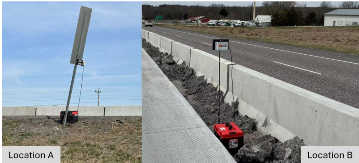
Figure 4-1. Sensor setup at the I-70 Kingdom City work zone.
