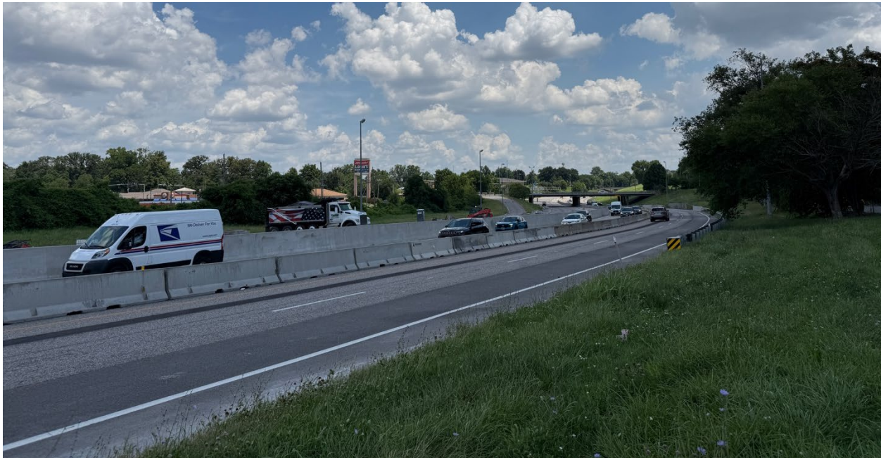
Figure 8-1. Two-way traffic separated by temporary barrier on I-55 in St. Louis.
