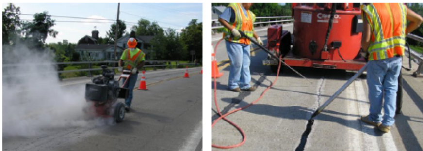
Figure A.3 Crack Sealing in Concrete Decks
