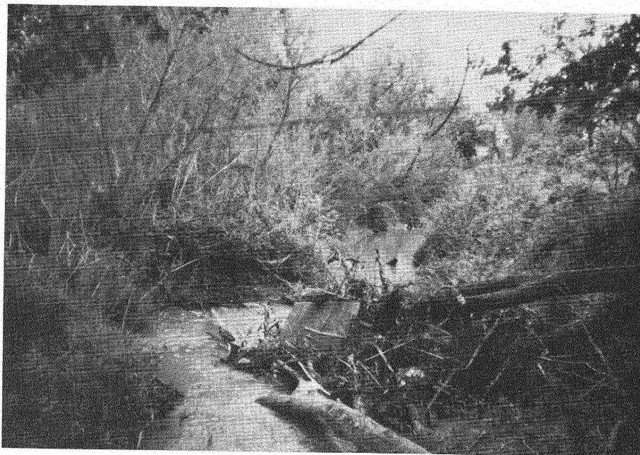
This photo depicts an ongoing problem which confronts ODOT. Willows which clog drainage ways and ditches will begin to collect debris, become unsightly and impede water flow.
