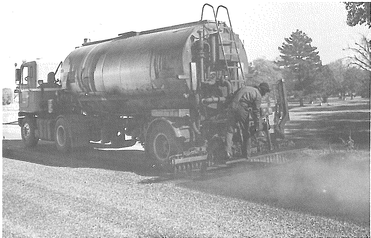
Figure 7. The application of asphalt-rubber by the modified distributor.
