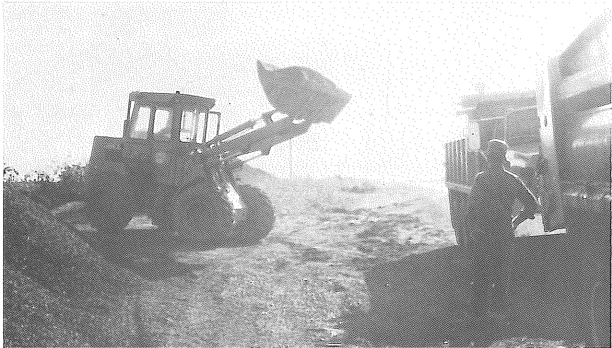
Figure 5. Loading the dump trucks with pre-coated aggregate.
