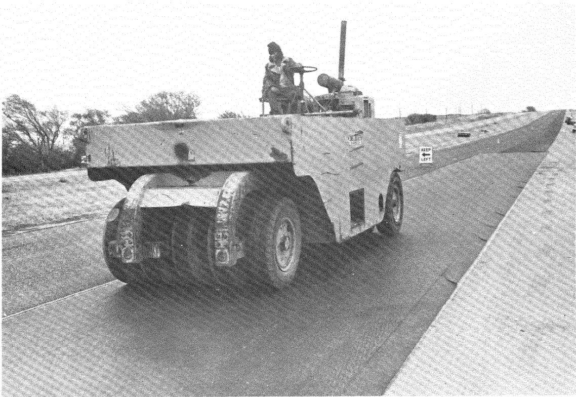
Figure 7 and 8. The recycled overlay was placed in a conventional manner. No special equipment was required.
