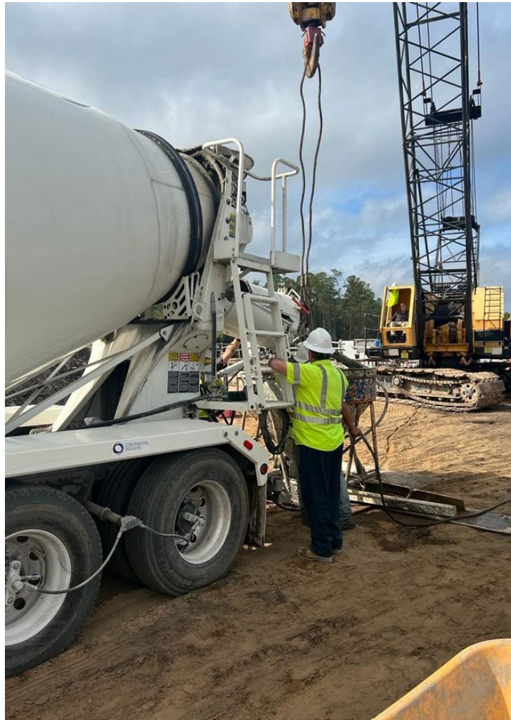
Figure 10. Placement of the first concrete mixture sampled
