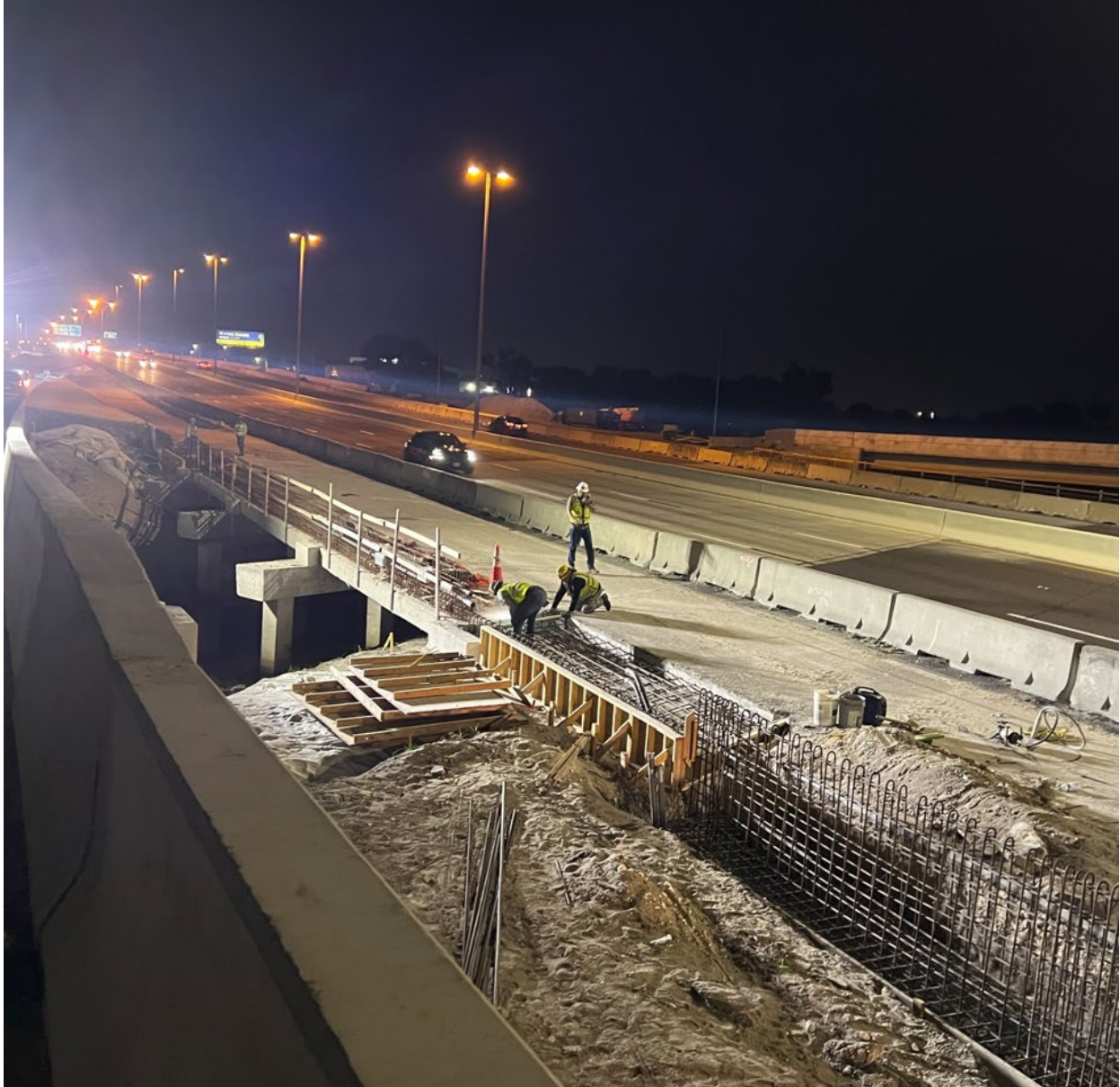
Figure 25. Construction site 8 placement
