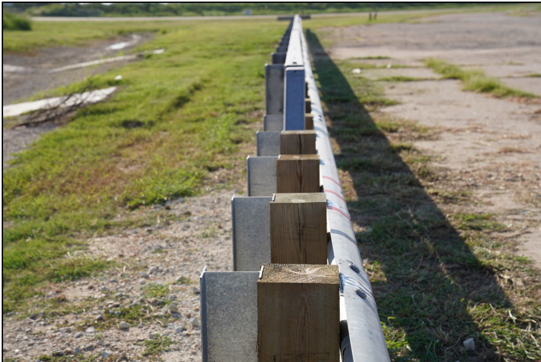
Figure 3.5. Upstream In-Line View of the Test Installation prior to Testing.
