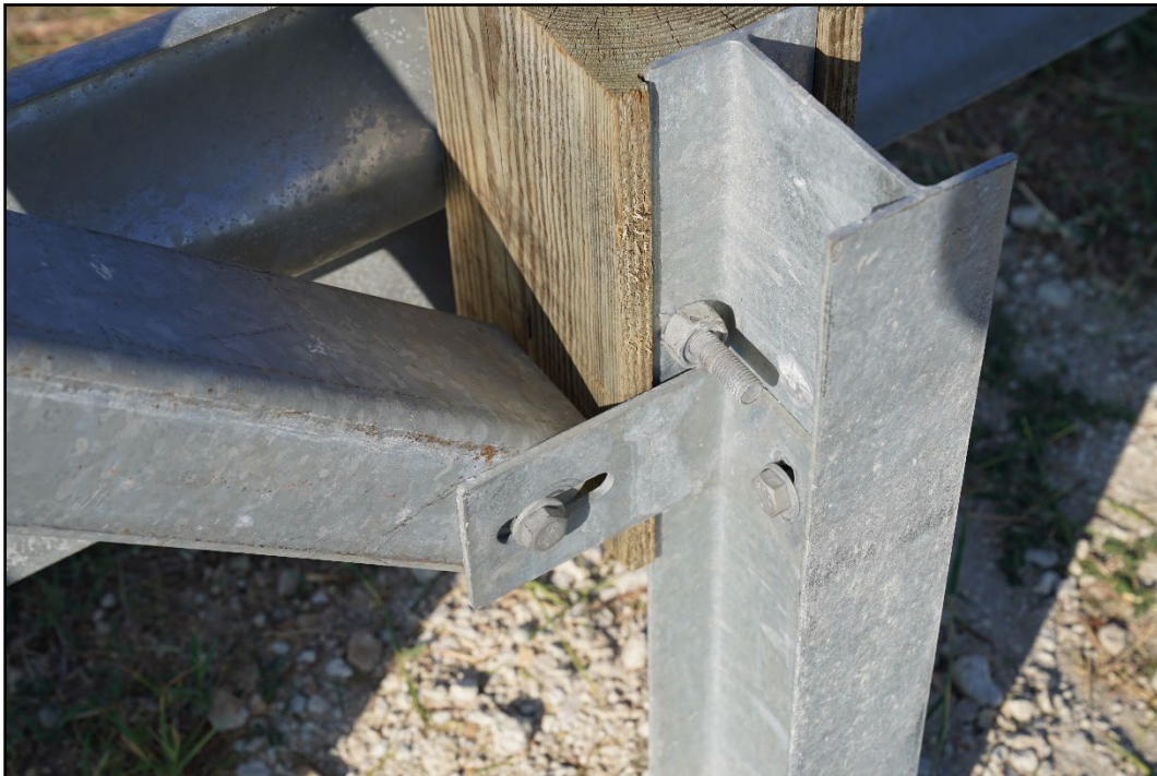
Figure 3.7. Transition Box Beam Rail Connection to Post 15 prior to Testing.
