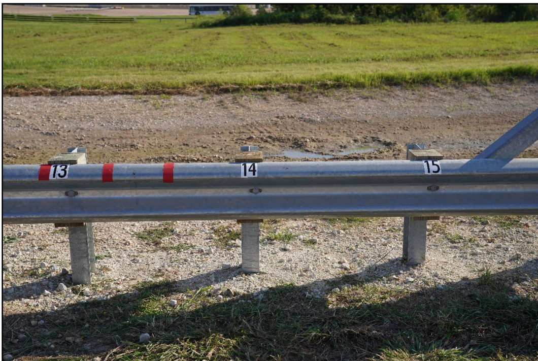
Figure 3.3. TL-4 Test Installation at Impact prior to Testing.
