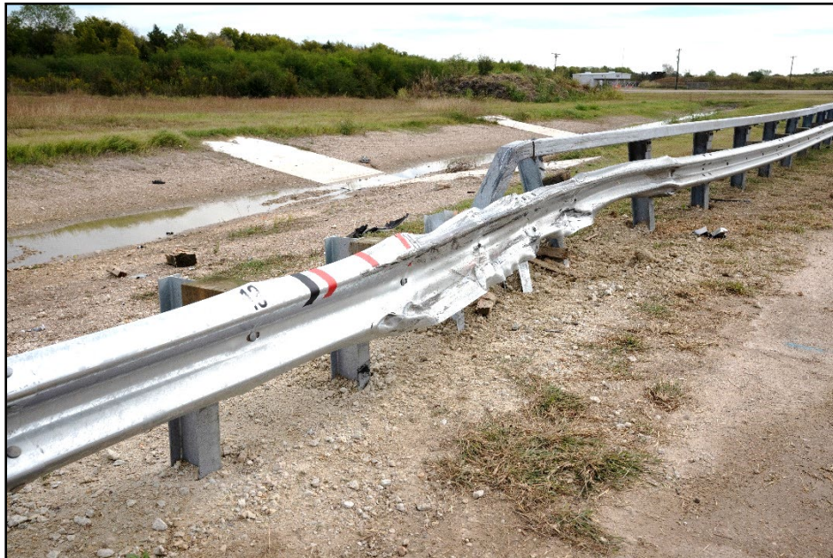
Figure 7.5. Transition at the Impact Location after Test 441203-01-2.
