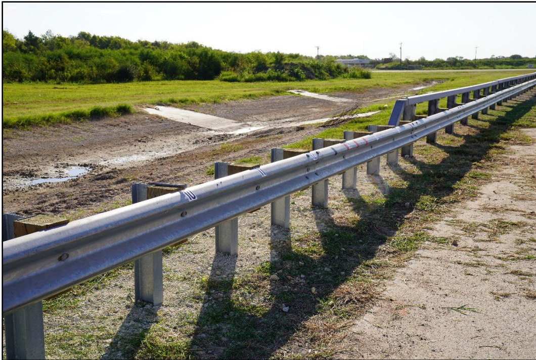
Figure 3.2. TL-4 Test Installation prior to Testing.
