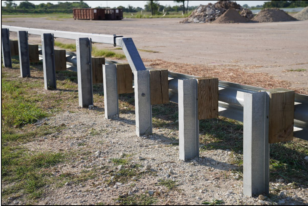
Figure 3.6. Field Side of the Transition prior to Testing.
