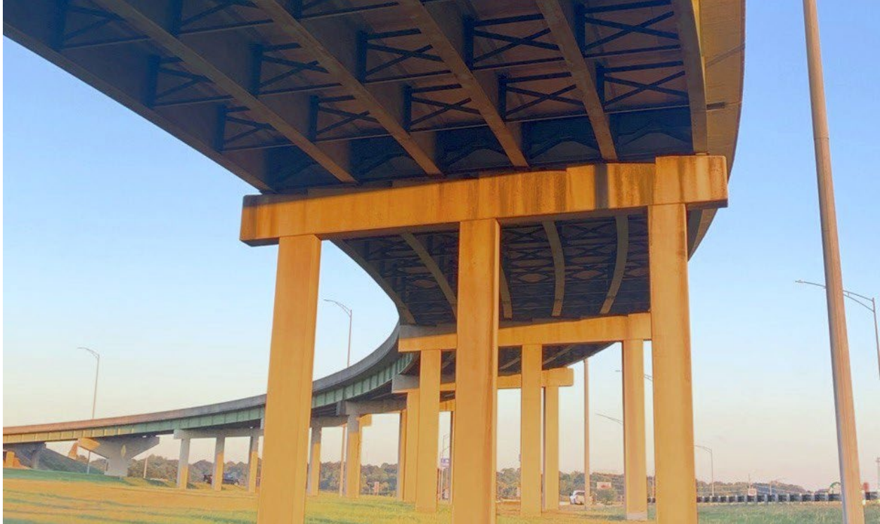
Figure 1-1. Curved steel I-girder bridge located in Tuscaloosa, Alabama, USA.
