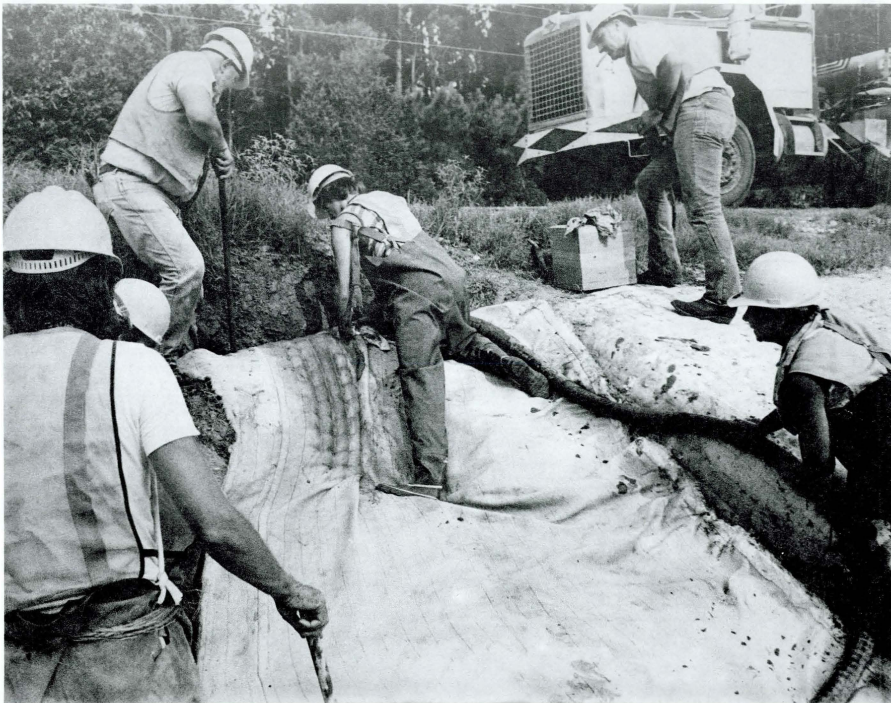
Figure 8. Filling Anchor Trenches.
