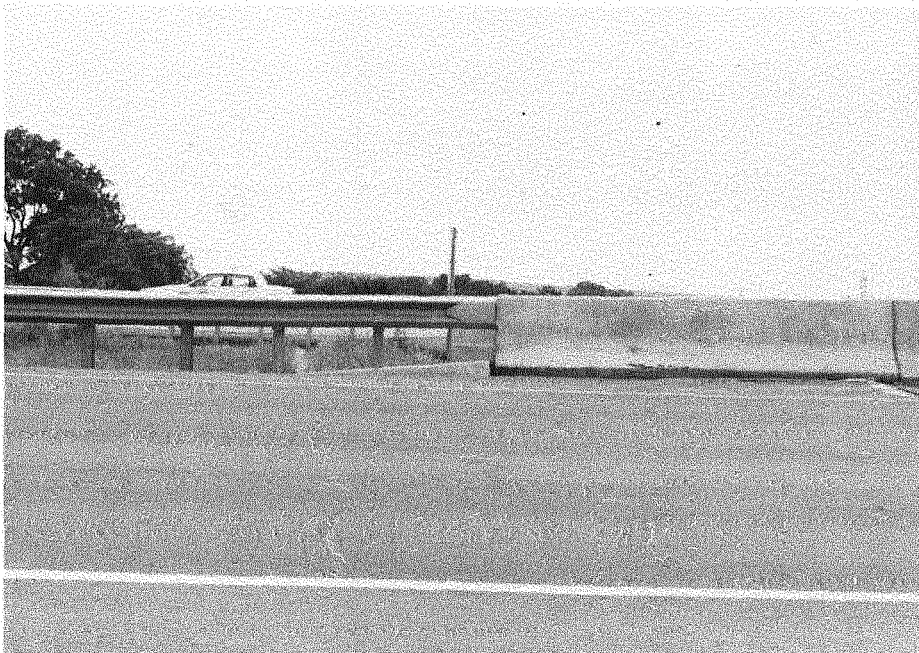
Fig. 2-3. Approach guardrail used since 1980
