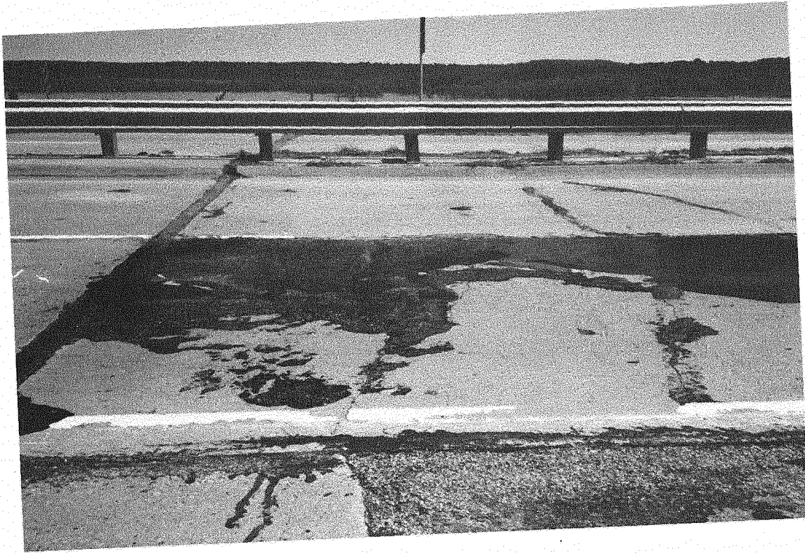
Fig. 2-8. A rough bridge approach
