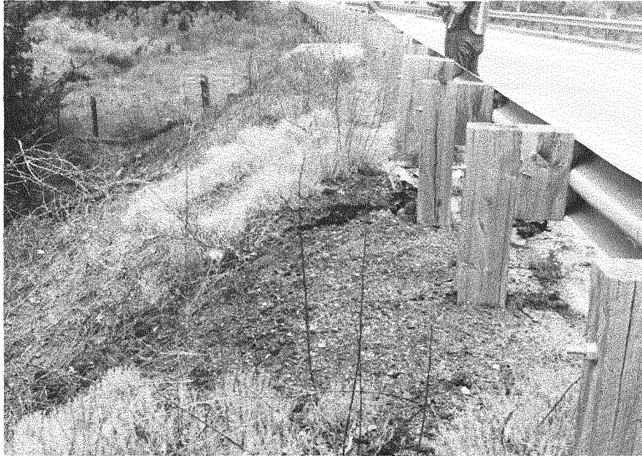
Fig. 2-2. Approach guardrail used during the period 1960-1980
