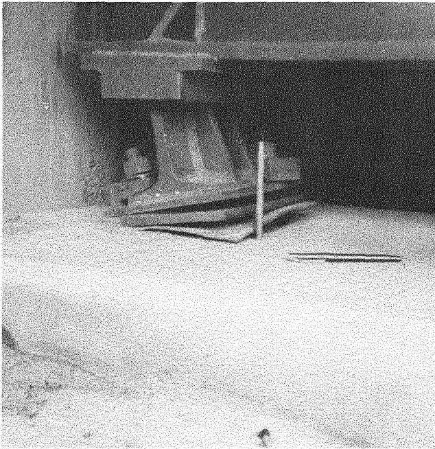
Fig. 2-21. Expansion device showing extensive tilting
