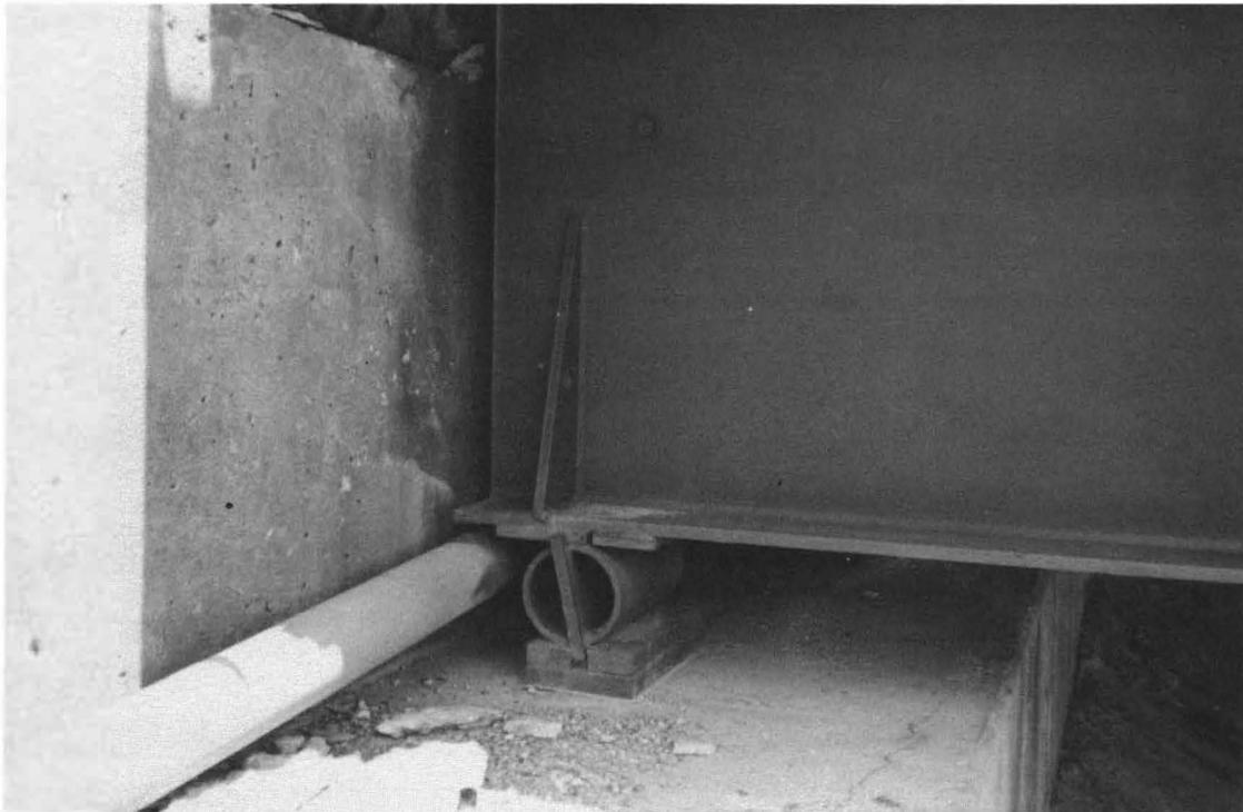
Fig. 3. An expansion device showing extensive tilting.
