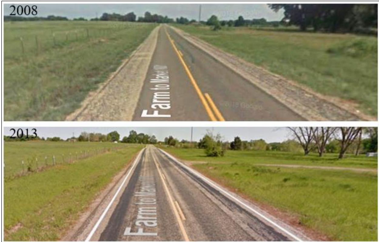
Figure 52. Existing (2008) and Widened Pavement (2013), Project 2.
