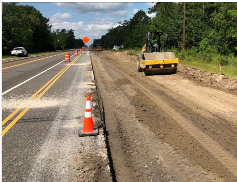
Figure 1. Pavement Widening in Beaumont District.
