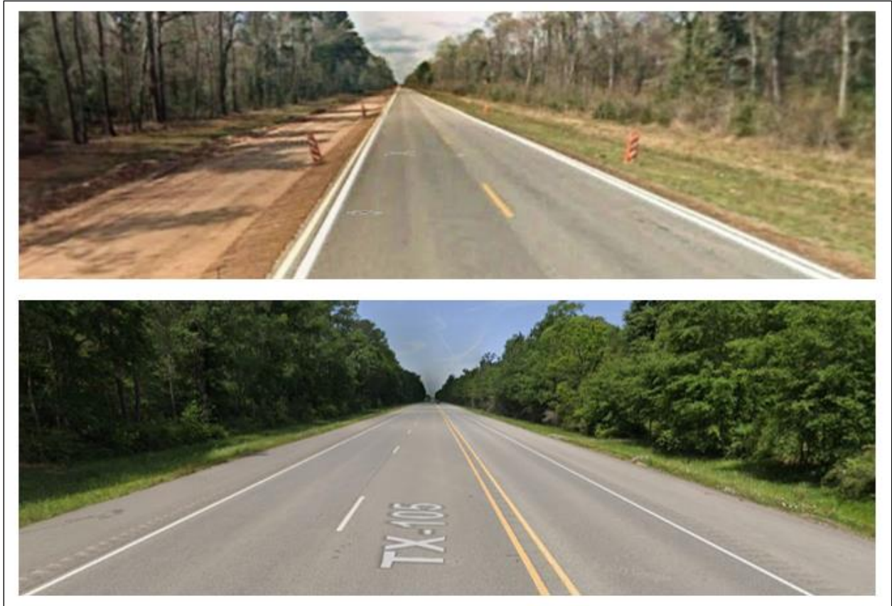
Figure 45. Construction (2008) and Current Pavement (2021), Project 1.
