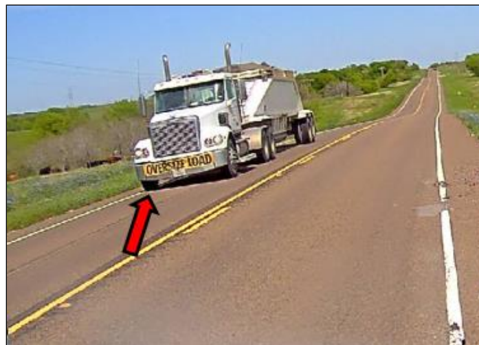
Figure 71. Traffic Tends to Drive near the Lane Edge and into the Widening, Project 4.
