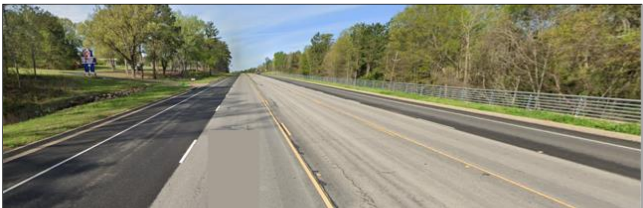
Figure 63. Repaired Outside Widened Lanes, Project 3.
