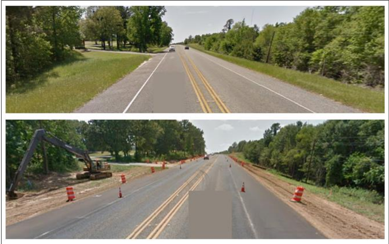
Figure 59. Existing Roadway and during Construction, Project 3.
