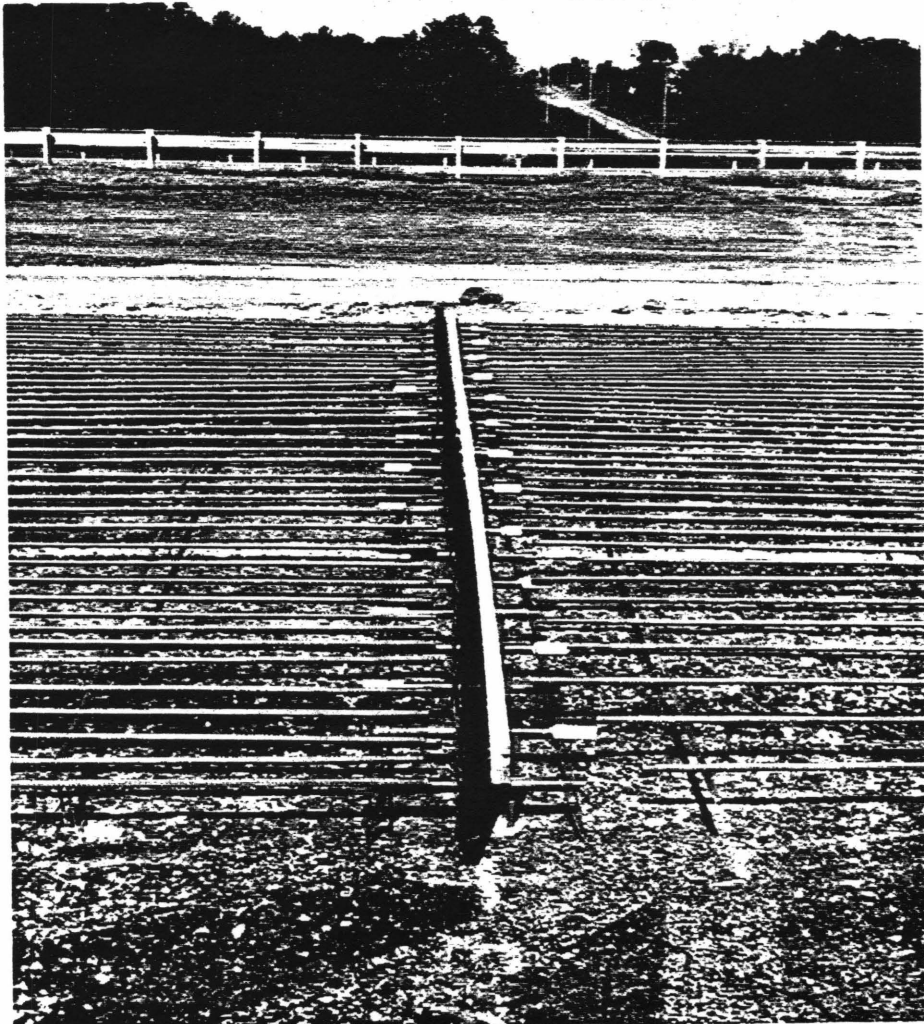
Figure 14. Dowel Bar Joint.
