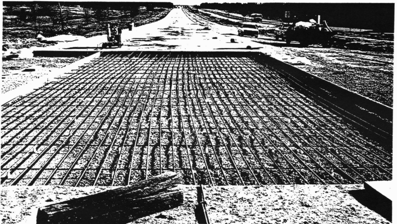
Figure 12. Preparing Remaining 60' Section for Paving.
