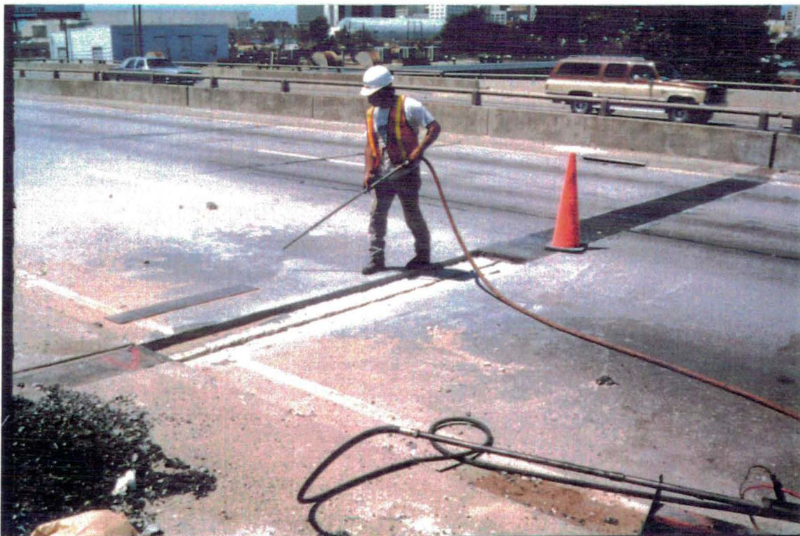
Figure 5. Heating Exposed Saw Cut, Expansion Gap, and Bridge Deck.
