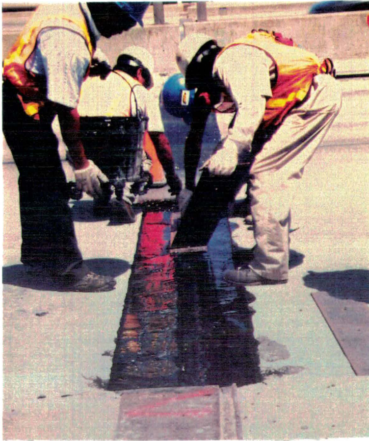
Figure 8. Placing Bridge Plate Over Sealed Expansion Gap.
