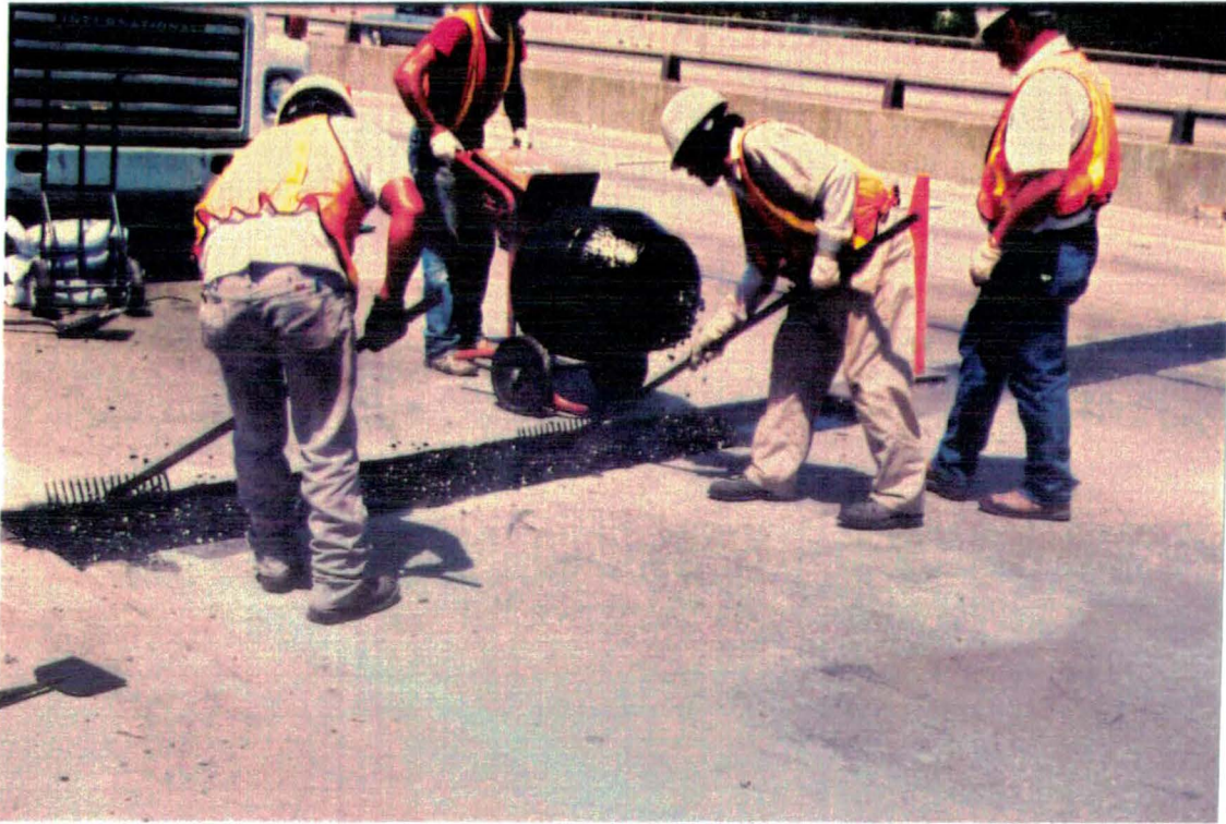
Figure 12. Placing 3/4 Inch Modified AC Mix.
