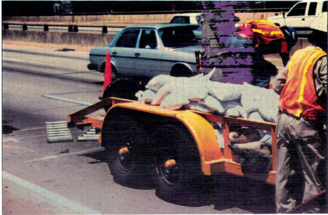
Figure 3. Bags of Granite Chip Aggregate.
