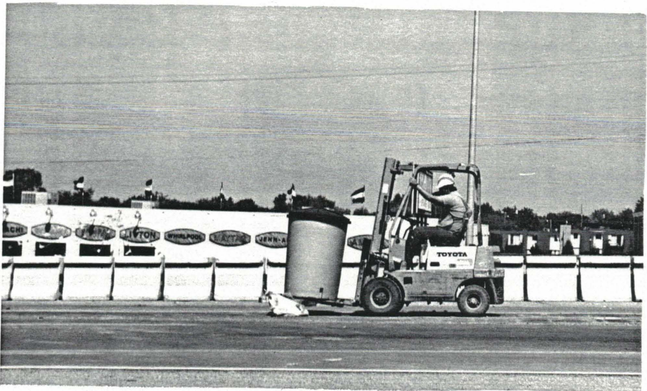
Figure 17. Moving End Protection Prior to Barrier Wall Shift.
