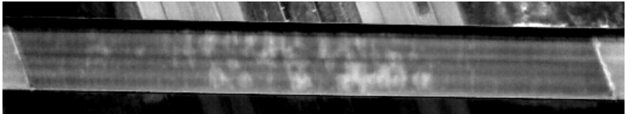
Figure 2 - B670122 - Drone Full Deck - 400 Feet Above Deck
