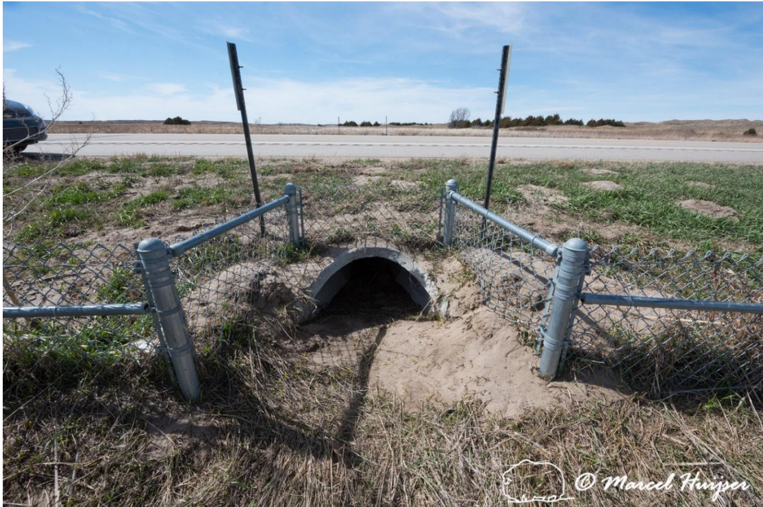
Figure 105. A chain-link turtle fence continues above a culvert for turtles, Valentine National Wildlife Refuge, Nebraska, USA.
