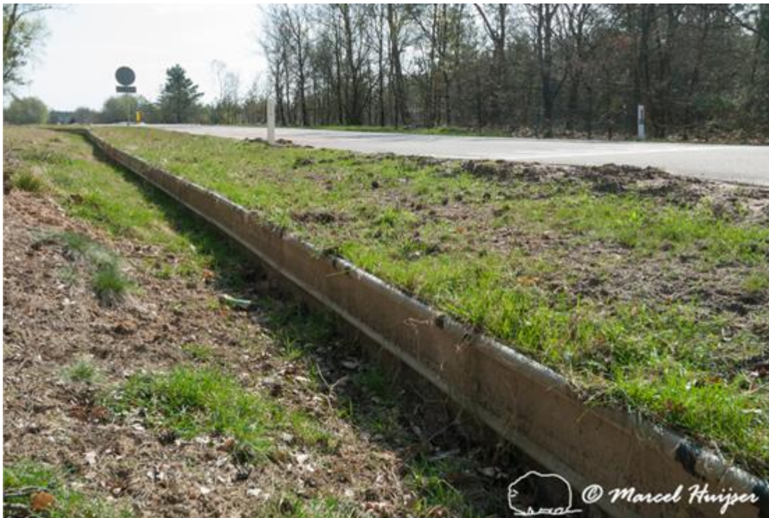
Figure 103. A “barrier wall” (polymer concrete) for common toads ( Bufo bufo ), integrated into roadbed, Deelenseweg, between Hoenderloo and Arnhem, Gelderland, The Netherlands.
