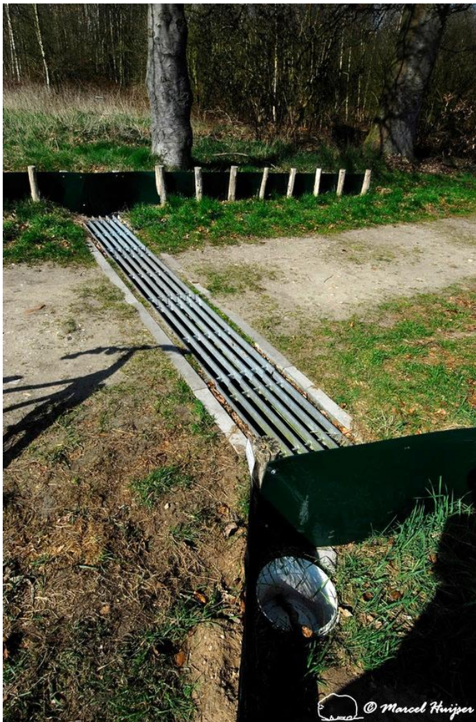
Figure 116. ABS plastic sheets to keep common toads off the highway (highway is to the left of the image), and an amphibian tunnel under an access road. Amphibians that approach the access road would fall in between the bars. Amphibians that travel along the barrier would go through the tunnel, continue to travel along the barrier on the other side of the access road until they encounter a tunnel that allows them to cross to the other side of the highway.
