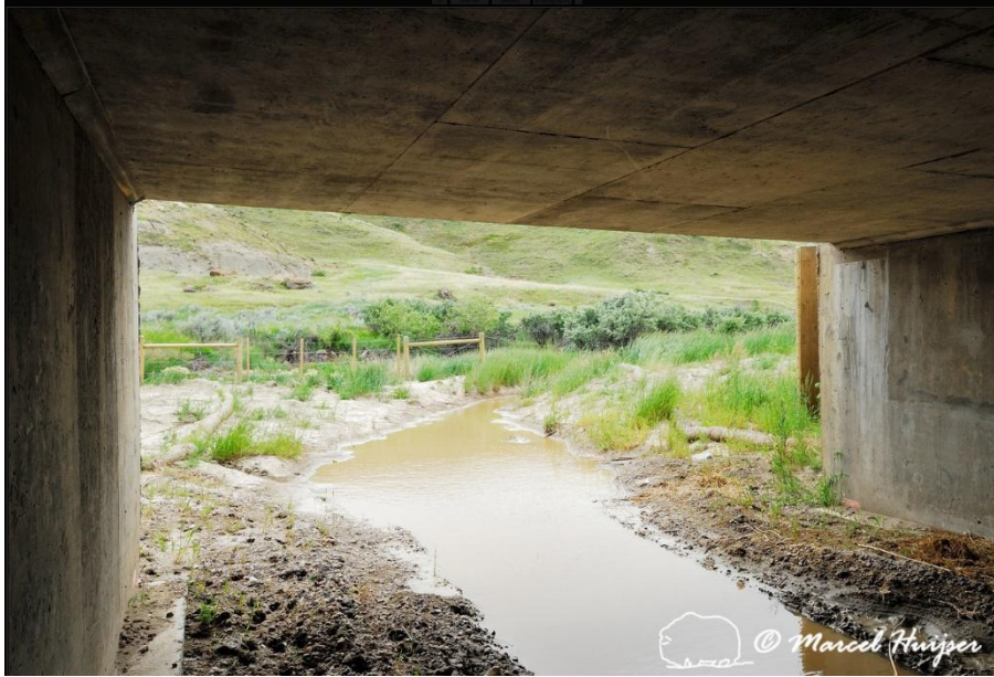
Figure 122. Bottomless culvert.
