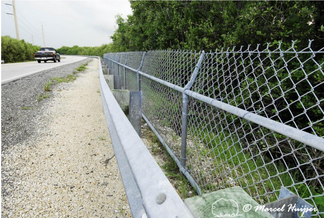
Figure 114. Fence with overhang for American crocodile ( Crocodylus acutus ), Key Largo, Florida, USA.
