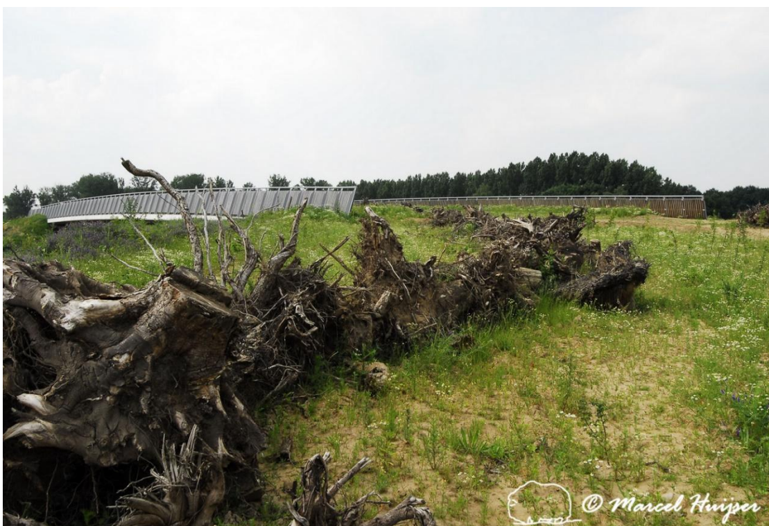
Figure 127. Root wads leading up to and on top of wildlife overpass as cover for small animal species, The Netherlands.
