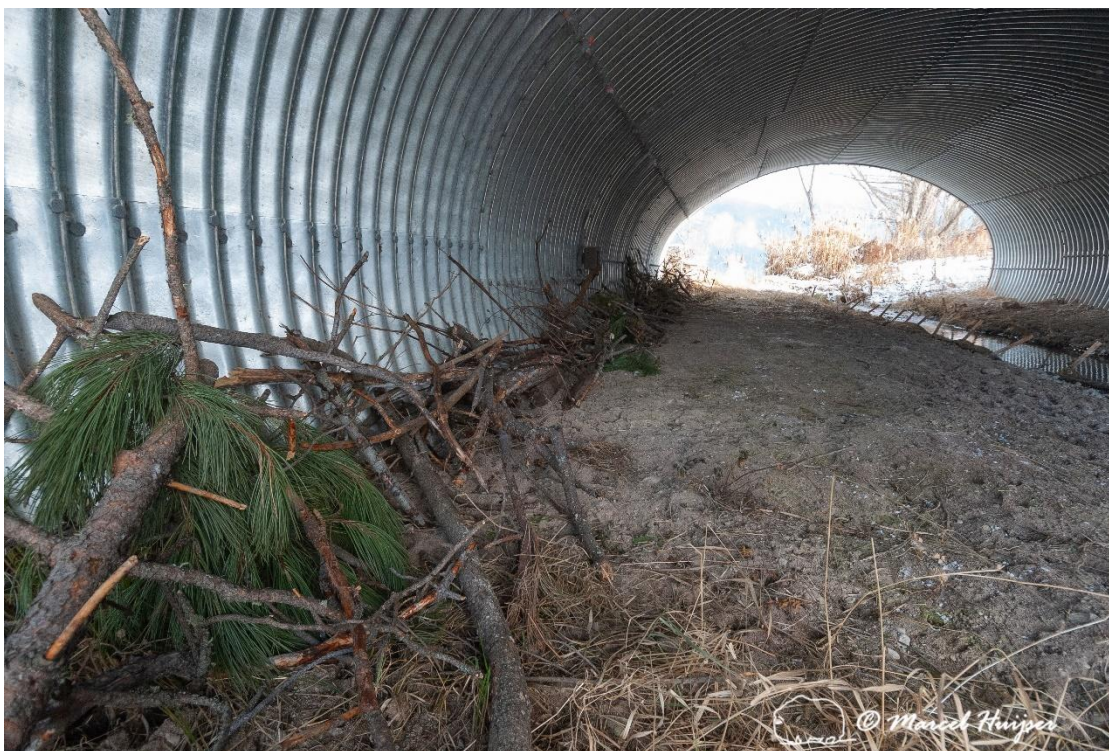
Figure 126. Wildlife underpass with branches along the side for cover for small mammals, Montana, USA.
