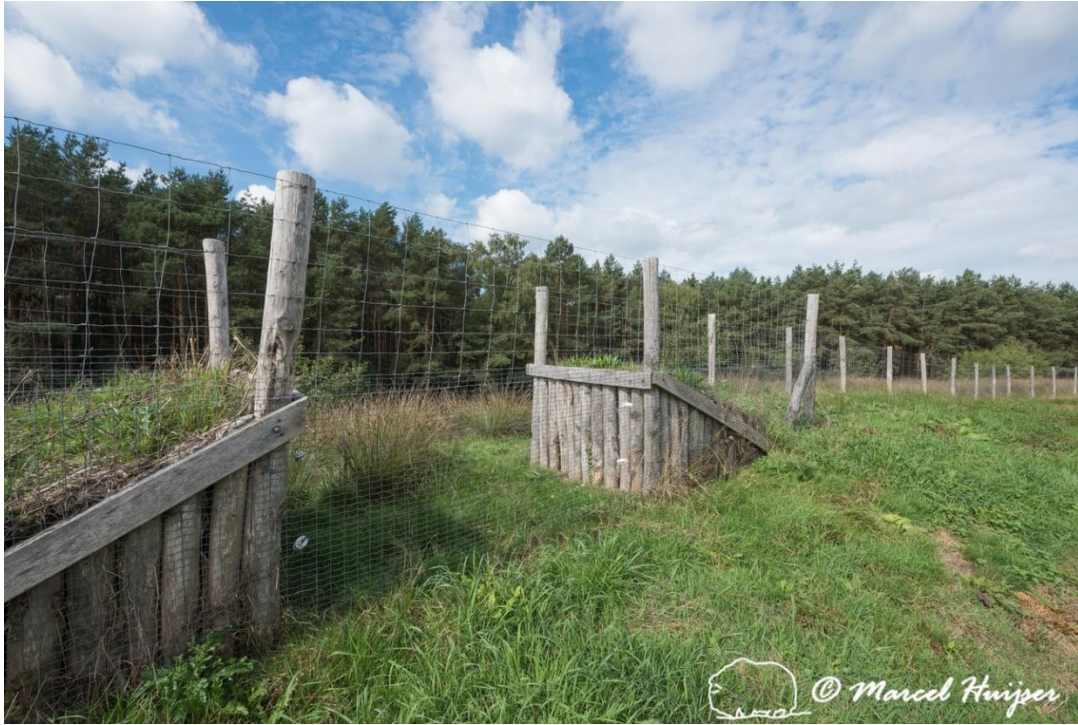
Figure 147. Wildlife fence and jump-out for medium sized mammals and roe deer, along A28 motorway, near Spier, Drenthe, The Netherlands.
