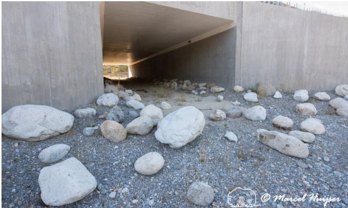
Figure 97. Boulders block access to unauthorized vehicles at wildlife underpass, US Hwy 95, Chilco, Idaho, USA.
