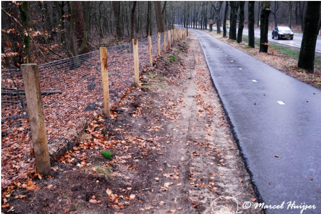
Figure 104. Wildlife fence for Eurasian badger ( Meles meles ) and wild boar ( Sus scrofa ), N302, Leuvenumseweg, Sonnevand, east of Harderwijk, The Netherlands.
