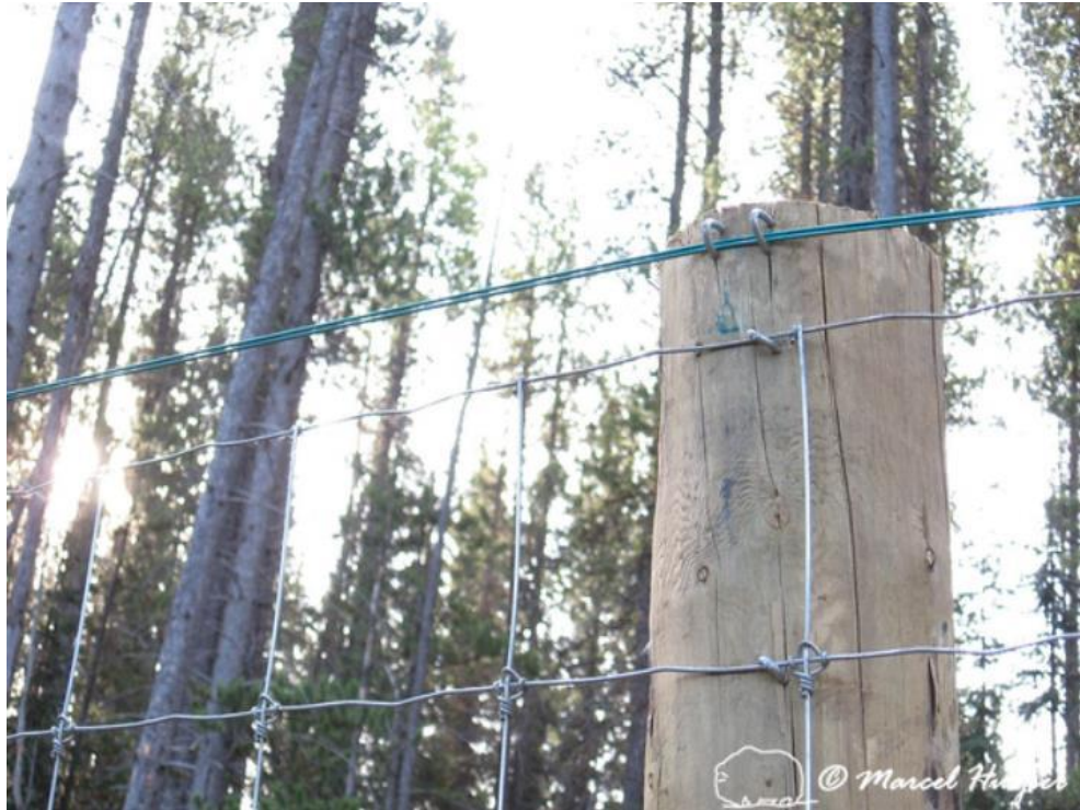
Figure 84. Wildlife fence with high-tensile top wire to reduce damage from falling trees, Trans-Canada Highway, Banff National Park, Alberta, Canada.
