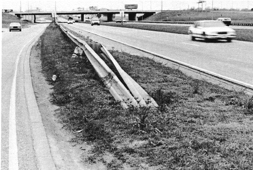
FIGURE 2.5 Double-faced turned-down end treatment
