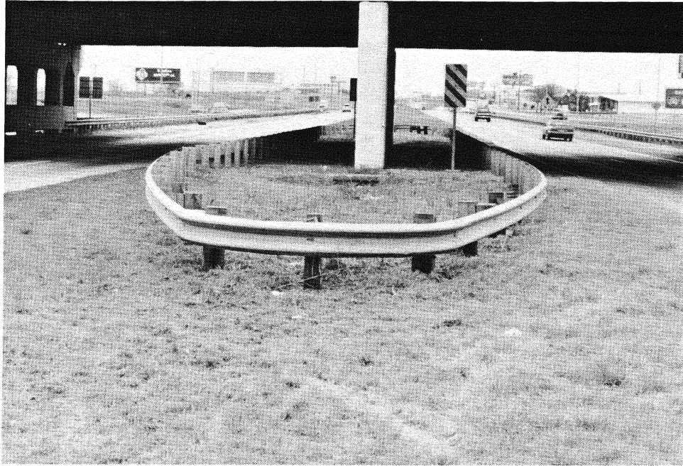
FIGURE 2.8 Parabolic end
