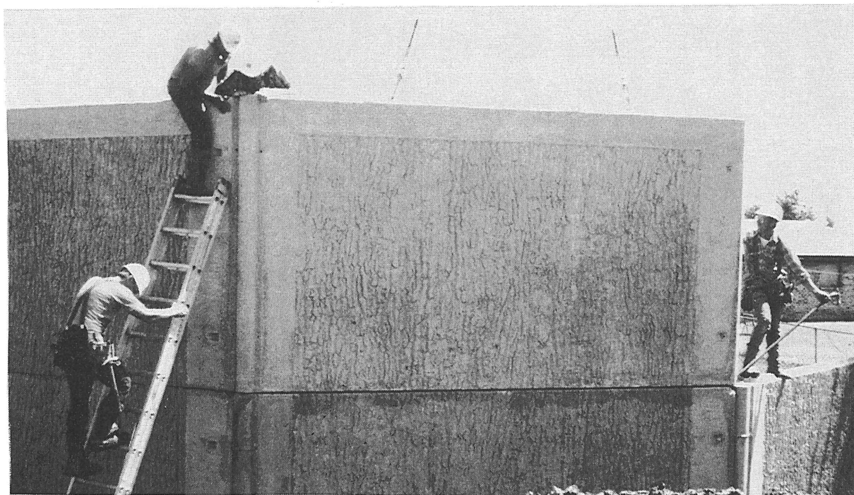
Figure 15. Guiding FANWALL Panels into Place.
