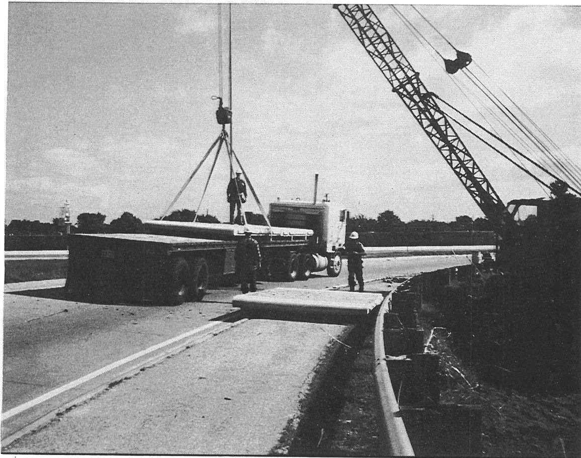
Figure 10. Unloading FANWALL Panel with Lifting Straps.
