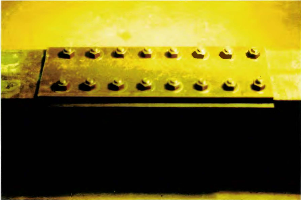
Figure 71. Splice Plate Detail
