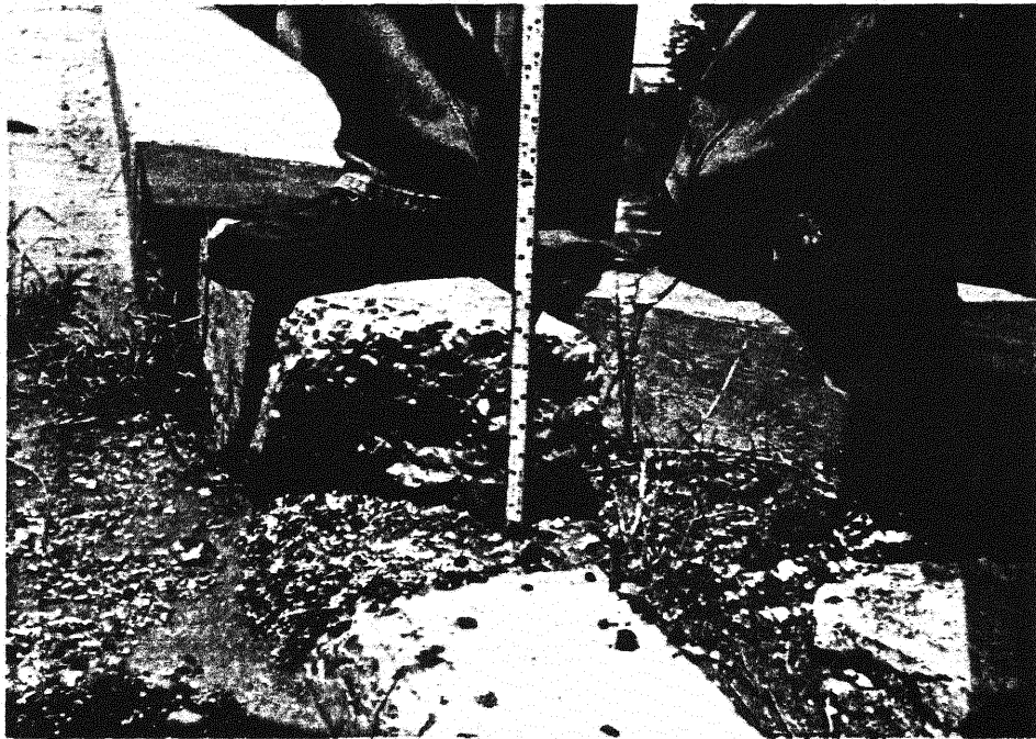
Fig. 2.1 Settlement estimate of bridge approach from the differential settlement of the curb.
