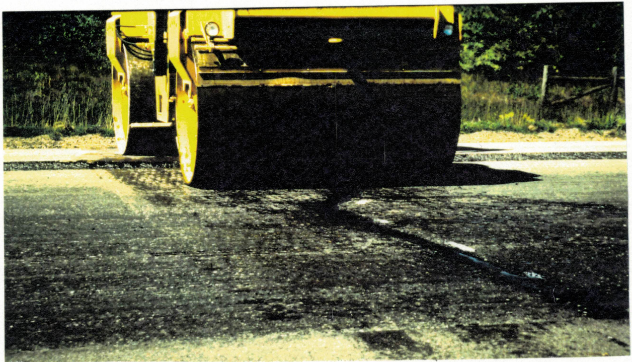
Figure 11. Rolling “Modified Type “B” Mix Used as Crack Patch Material.
