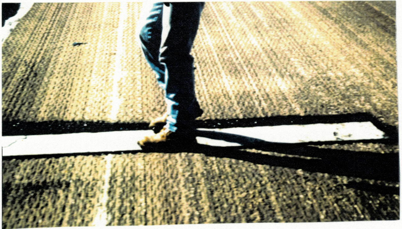
Figure 13. Pressing Pro-Guard into AC-20.
