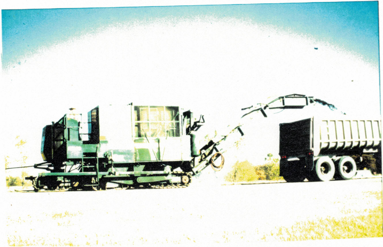
Figure 7. Coldmilling, Project NH-186(190)
