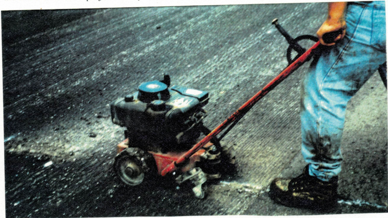
Figure 9. Routing Cracks.
