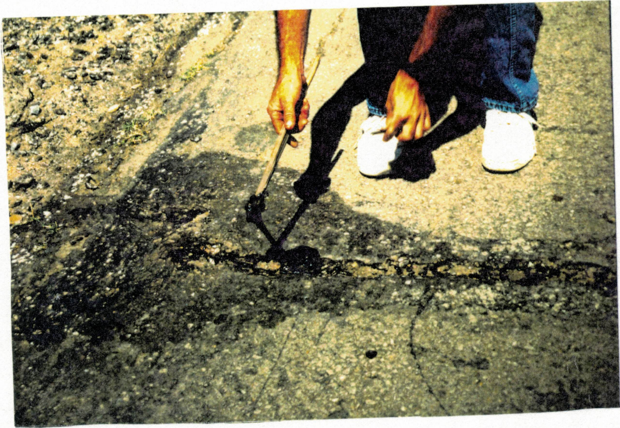
Figure 4. Uncured CRS-2 in Cracks.
