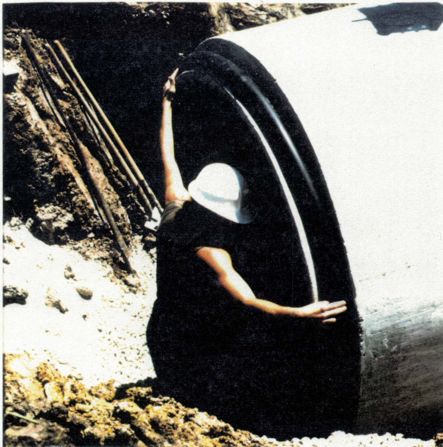
Figure 1. Placing Omni-Flex Seal on RCP section.
