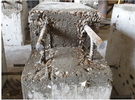
Figure 2.16: Exposed Aggregate Look of Base Blocks
