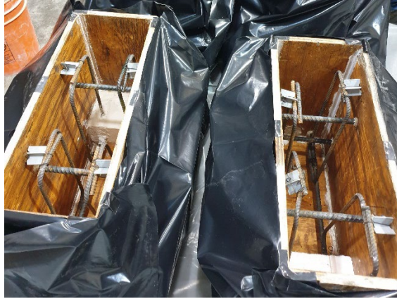
Figure 2.15: Base Blocks Formwork
