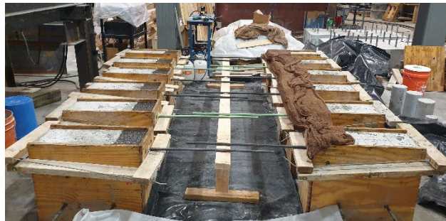
Figure 2.17: UHPC Bond Block Formwork
