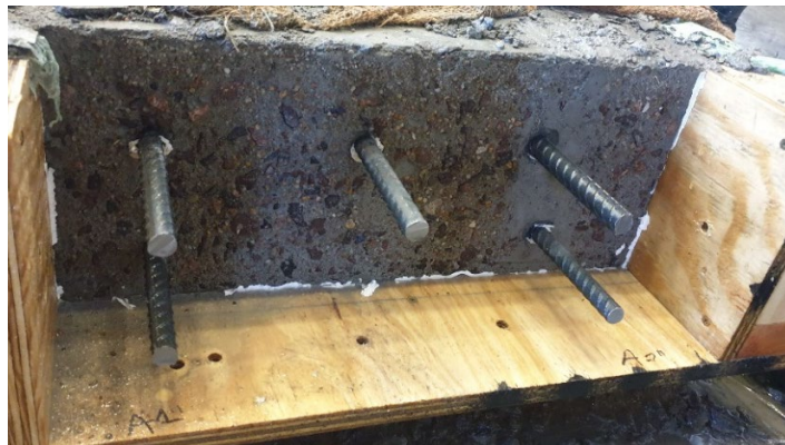
Figure 2.20: Exposed Aggregate Look of Side Panel
