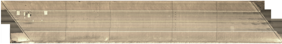
Figure 31 Overall View Images of Bridge Deck No. 22451
