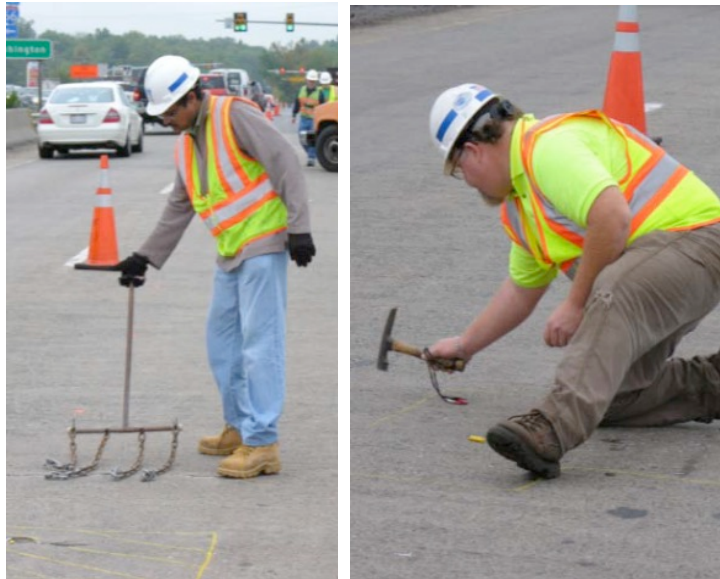
Figure 13 Chain Dragging and Hammer Sounding Technique [6]
