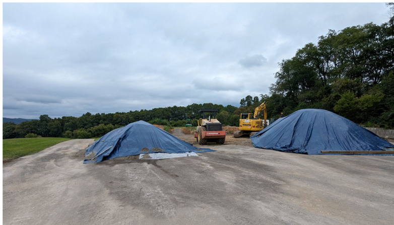
Figure 4-11. Water-proof plastic sheets protecting aggregates in SD condition from incoming storms or overnight precipitation.
