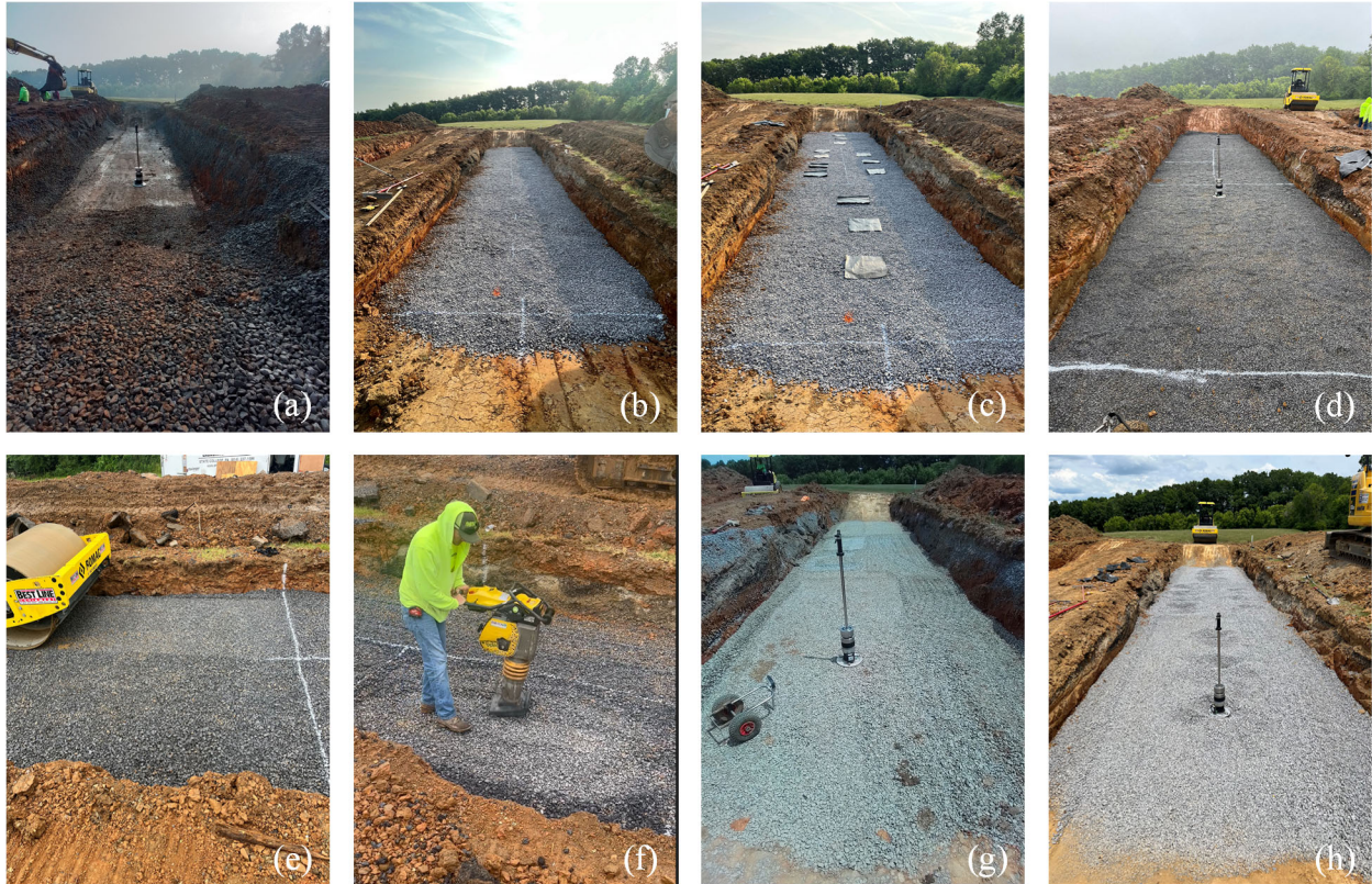
Figure 4-13. Photos taken during field tests: (a) LWD testing of trench bottom; (b) placement of aggregate to half of lift thickness and mark LWD test locations; (c) placement of geotextile fabric at LWD test locations at half of lift thickness; (d) LWD testing of uncompacted surface after placing 1 st lift; (e) aggregate compaction using the smooth single-drum vibratory roller (7.5 ton); (f) aggregate compaction using the hand impact rammer; (g) LWD testing of compacted surface; (h) LWD testing of mid-depth of lift on exposed geotextile fabric surfaces.
