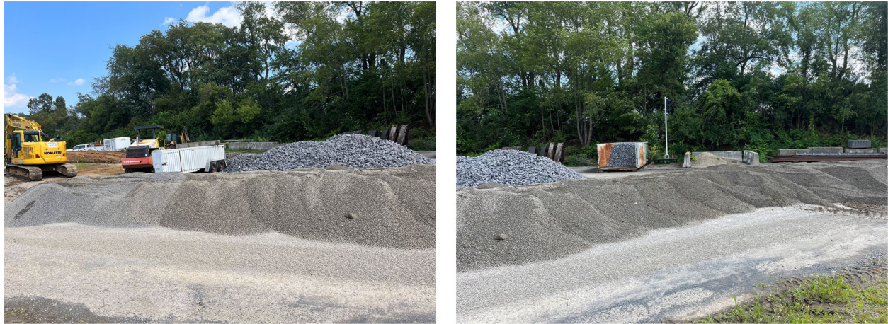
Figure 4-12. Aggregates in SS condition were spread out to expedite drying.
